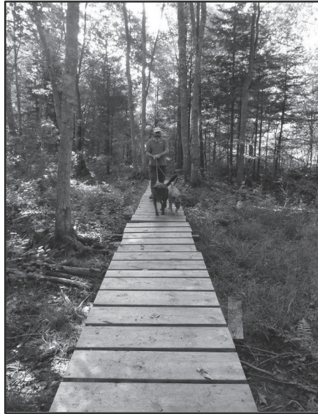
Putting the new boardwalk to use!
