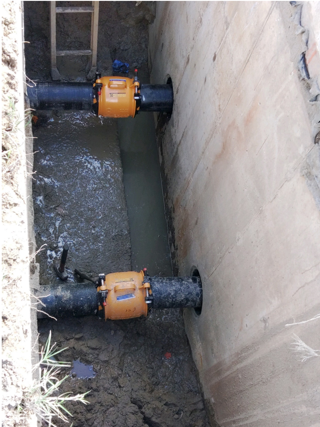
Repairs made to pumps #1 and 2 discharge pipes
