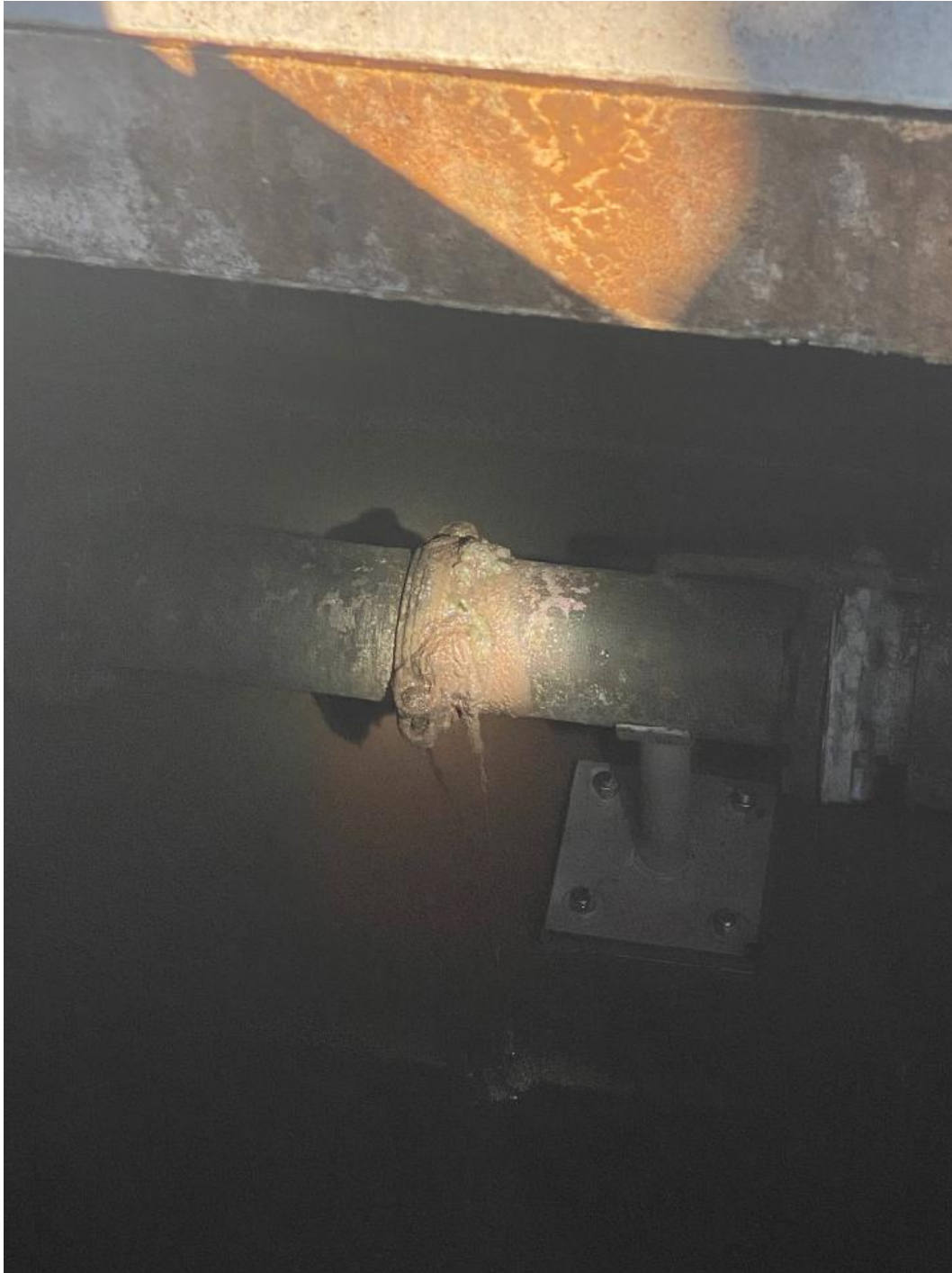
Pipe found on October 4, rags sealing the hole
