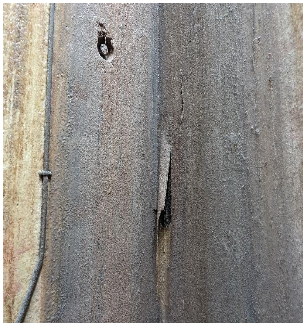
Lift Station - Failed Wall Coating
