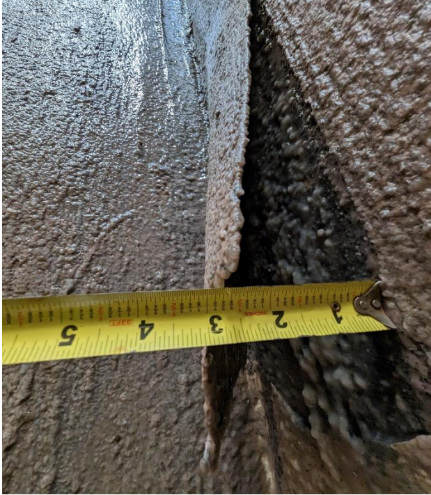
Lift Station - Protruding Coating Measurement
