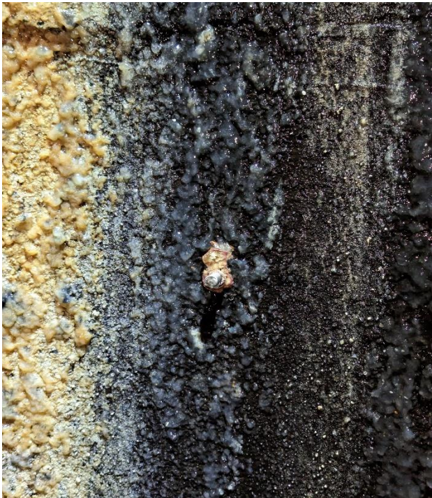
Old Wet Well - Exposed Anchor Bolt
