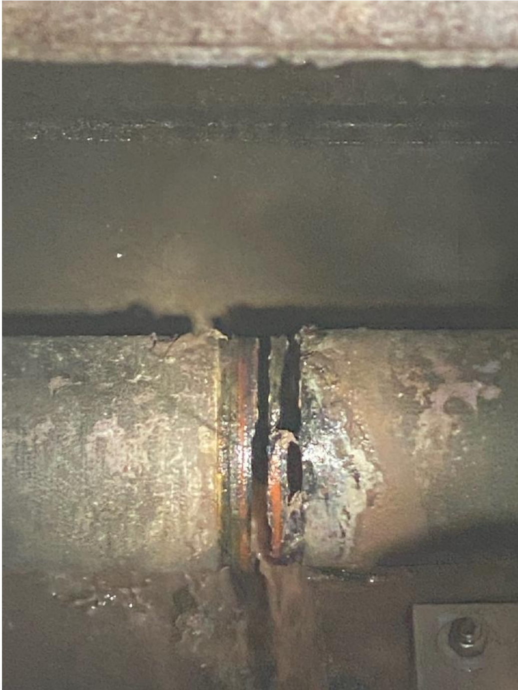
Pipe after coupling and rags removed, this is the pipe after all three pumps merge into one pipe
