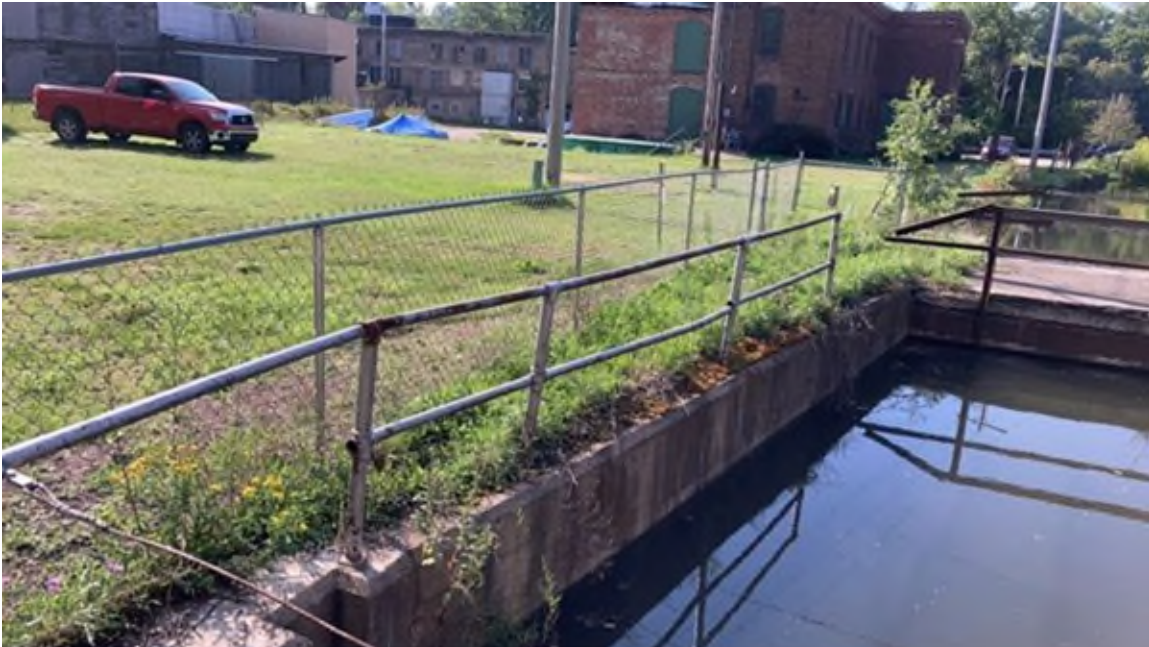
Photo #15 - Upstream slope of left embankment near powerhouse, vertical concrete millrace wall
