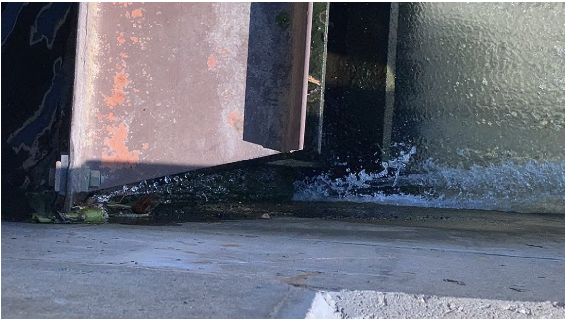
Photo #104 - Minor leakage on right side of spillway bay #3 gate
