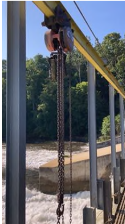
Photo #87 - Lifting mechanism for stoplogs of bay #2
