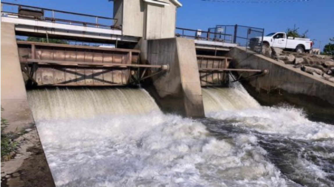
Photo #97 - Downstream view of two radial gate bays
