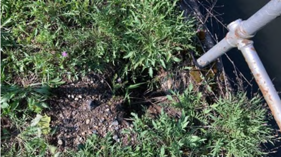
Photo #51 - Burrow or sinkhole on left embankment adjacent to millrace
