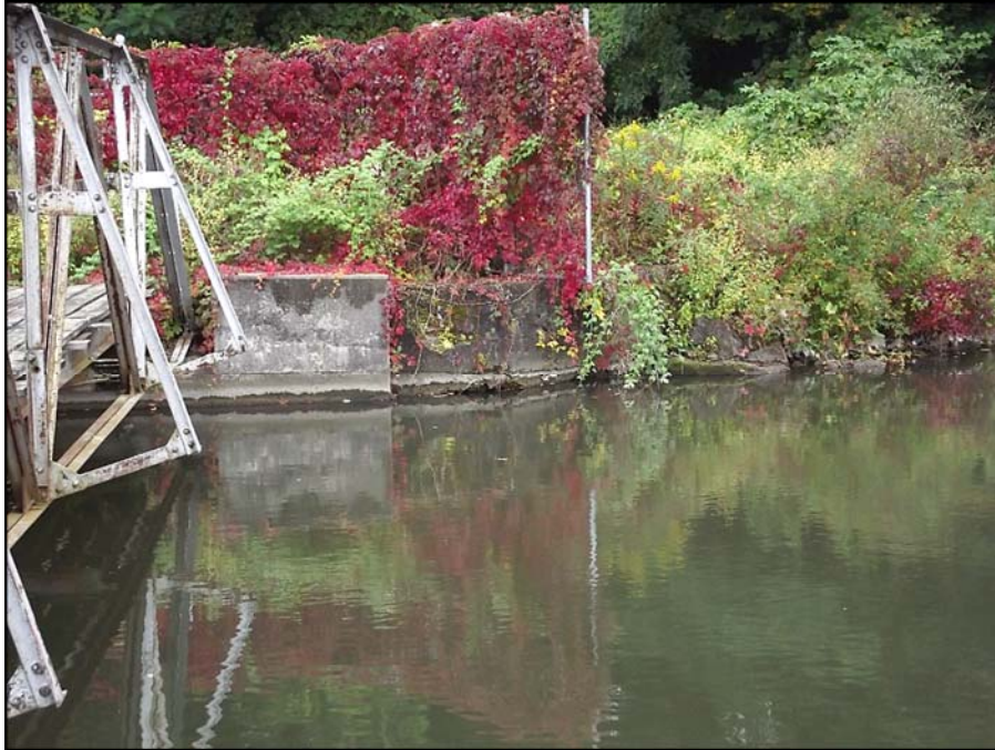
Photograph 11 – Upstream right abutment wall Note the overgrowth of vegetation and spalled concrete
