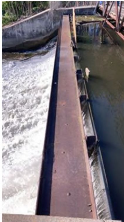
Photo #72 - Spillway bay #1, very slight deflection in beam over crest
