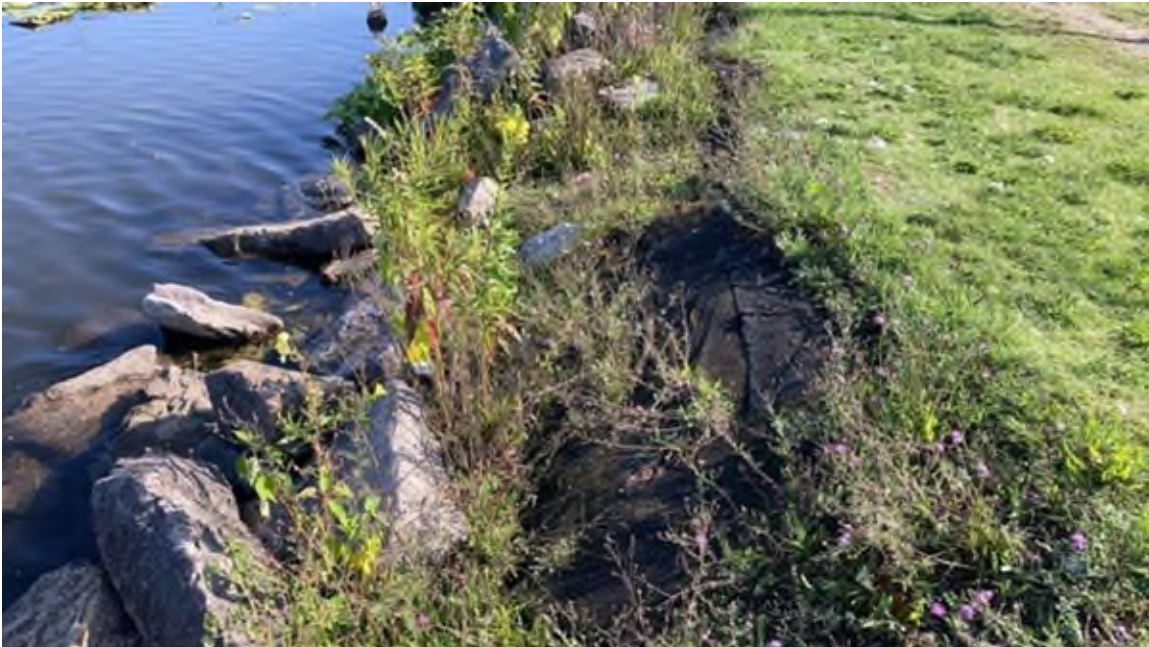
Photo #11 - Upstream slope of left embankment near spillway. Note exposed fabric where riprap is displaced
