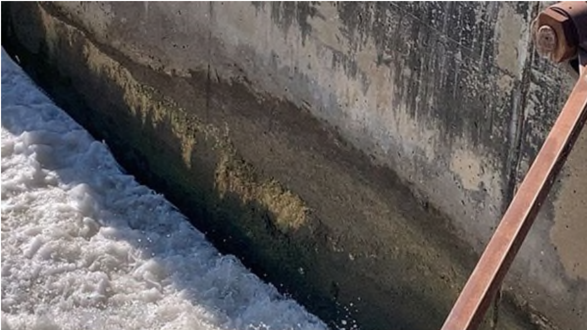
Photo #111 - Minor spalling on spillway bay #3 right downstream side
