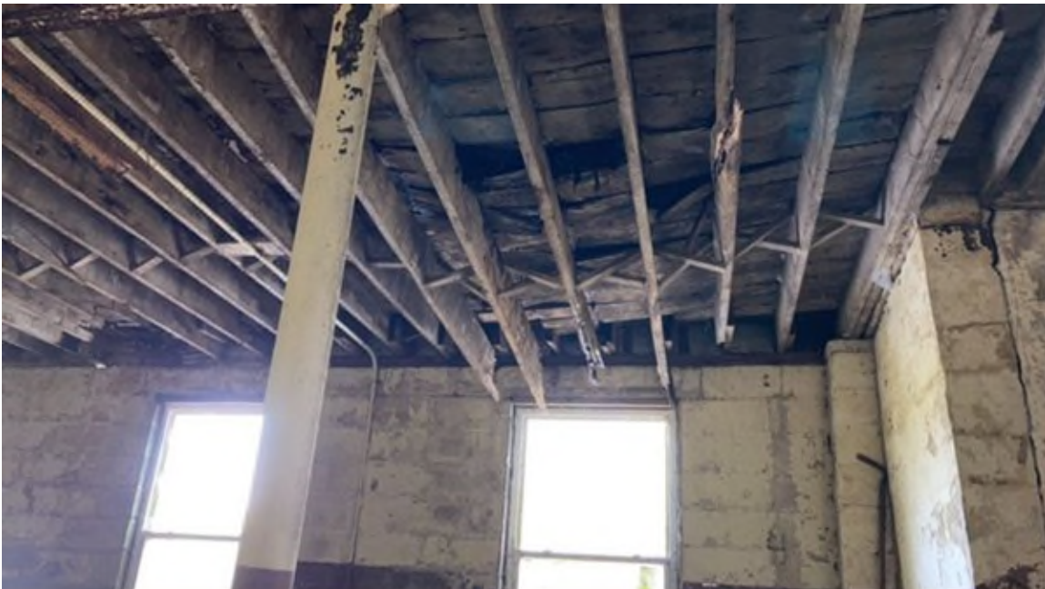
Photo #156 - Failing ceiling on left side of powerhouse
