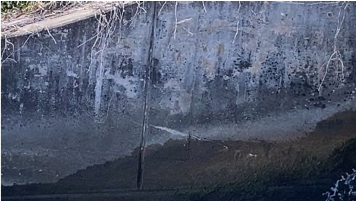
Photo #76 - Spillway right downstream abutment wall joint
