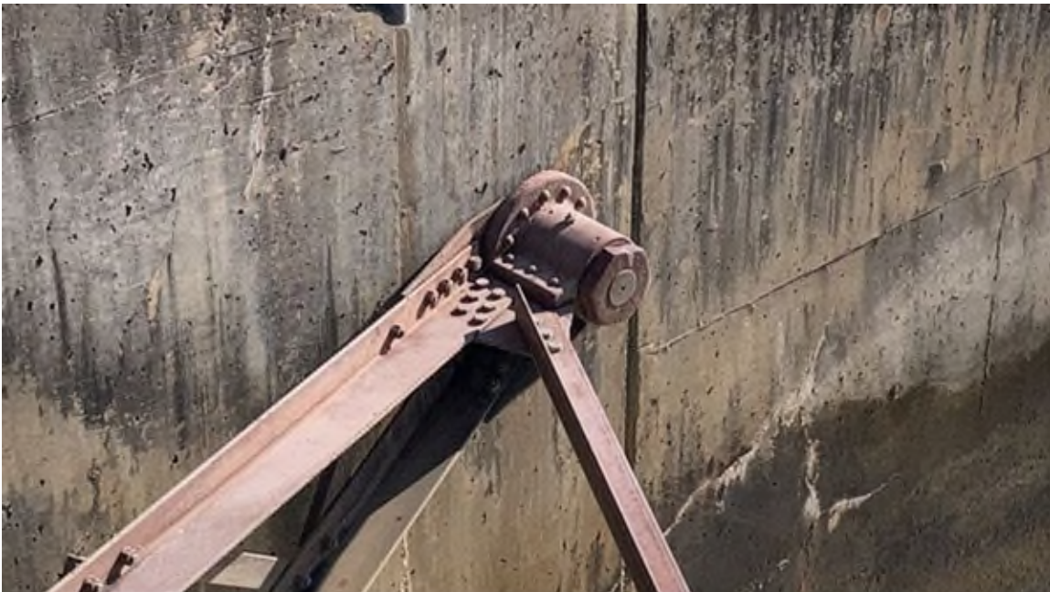
Photo #122 - Spillway bay #4 gate's left pin
