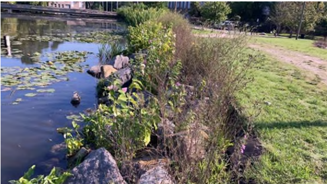
Photo #12 - Upstream slope of left embankment. Note brush near waterline
