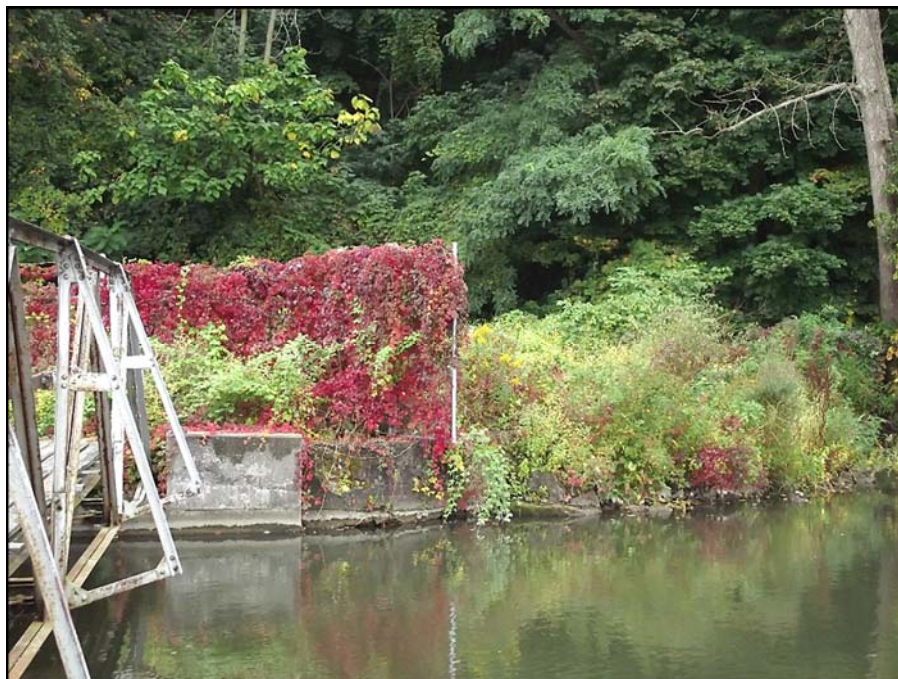
Photograph 7 – Upstream face of right embankment viewed from left Note that deterioration of the catwalk prevents access
