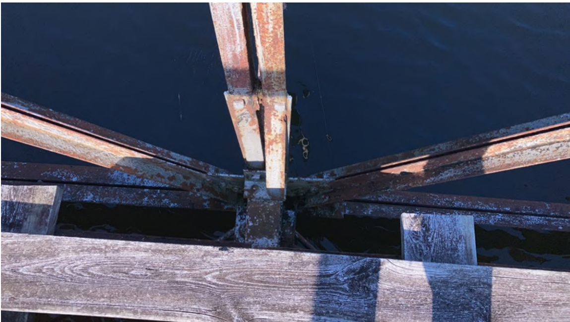
Photo #70 - Typical walkway bridge truss connection
