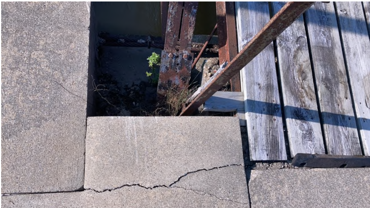
Photo #86 - Left end of walkway bridge, cracking concrete
