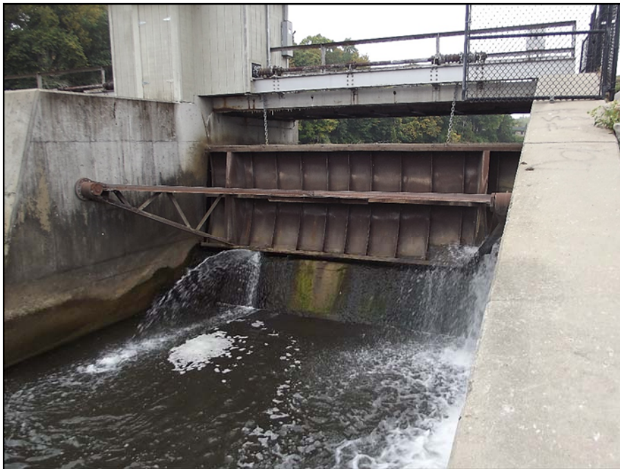
Photograph 22 – Typical radial gate viewed from downstream
