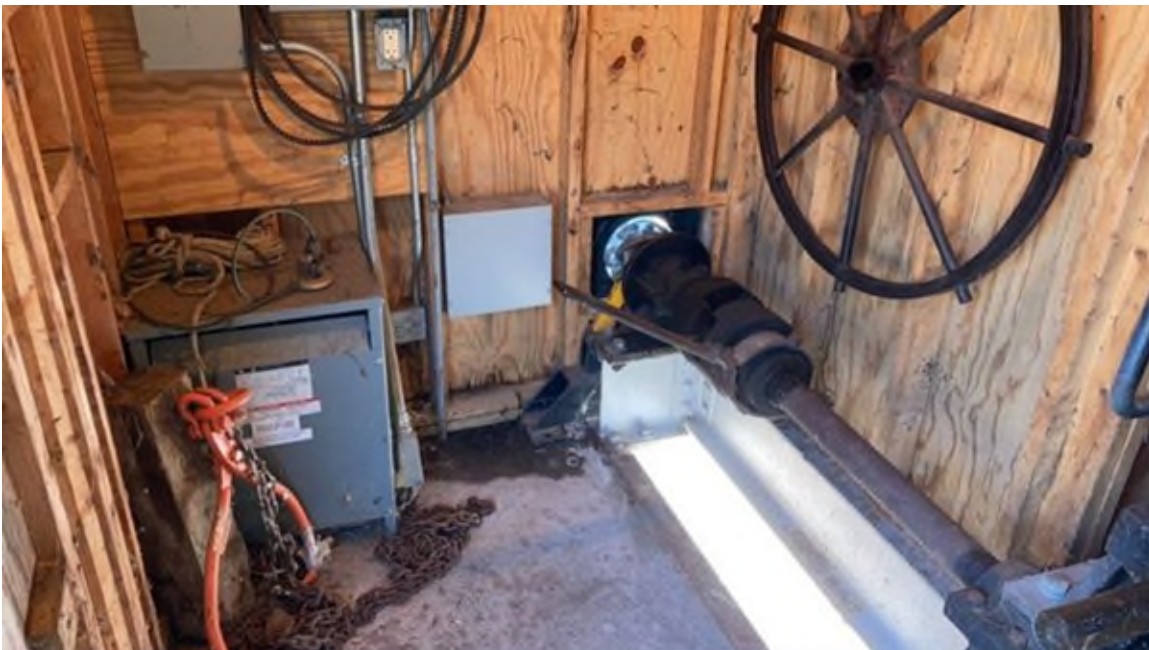
Photo #114 - Radial gate lifting shaft
