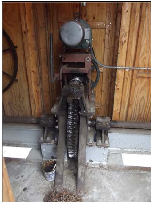
Photograph 24 – Radial gate operator
