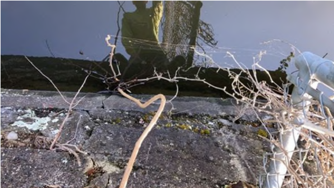
Photo #53 - Spillway right upstream abutment wall. Note concrete deterioration
