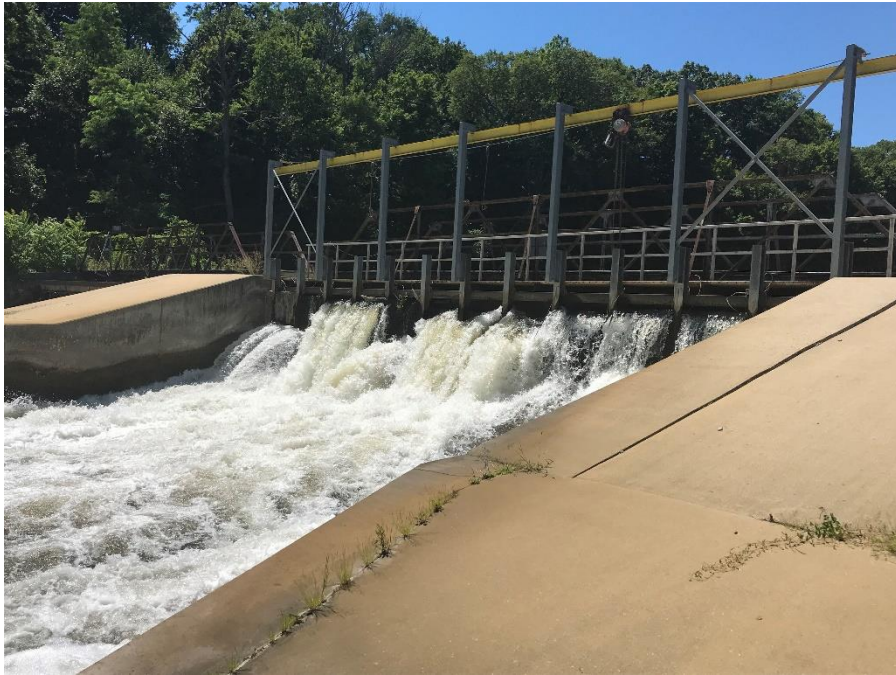
Photograph 19 – Center stoplog spillway viewed from downstream
