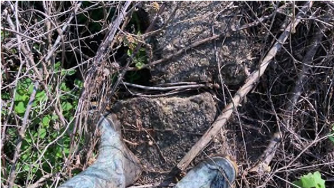
Photo #55 - Spillway right upstream abutment wall. Note concrete joint displacement
