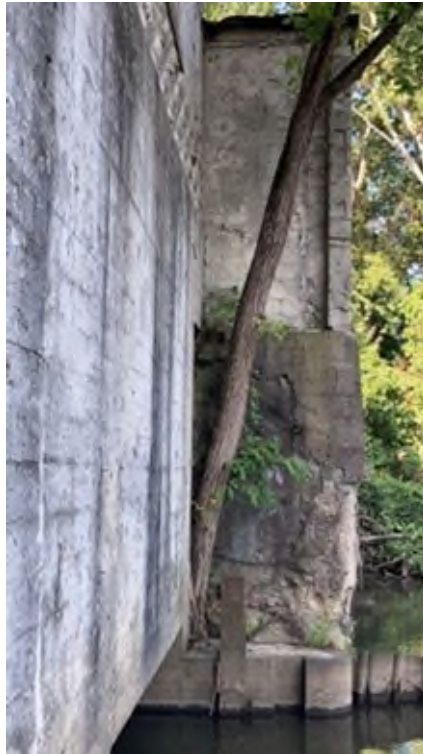
Photo #149 - Downstream face of powerhouse. Note tree growing between old and new portions of powerhouse
