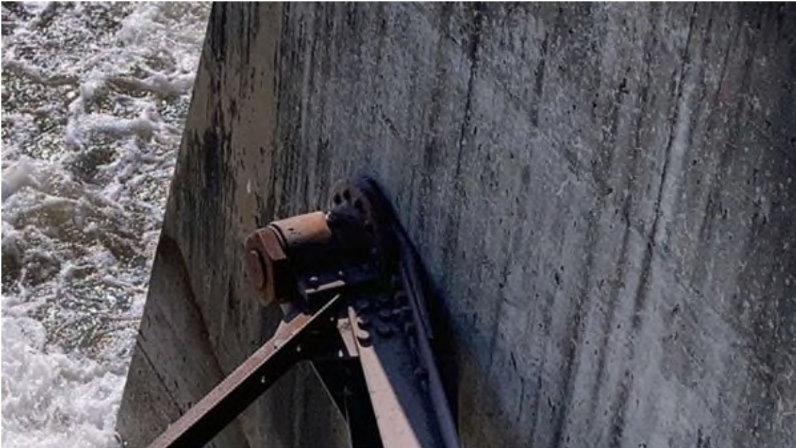
Photo #121 - Spillway bay #4 gate's right pin
