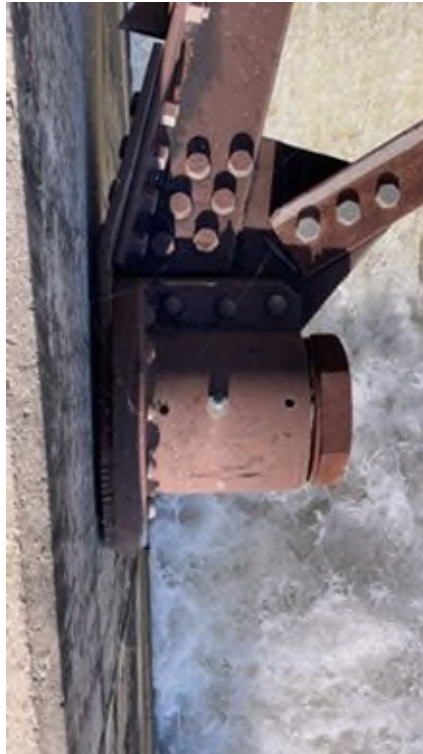
Photo #105 - Spillway bay #3 right pin
