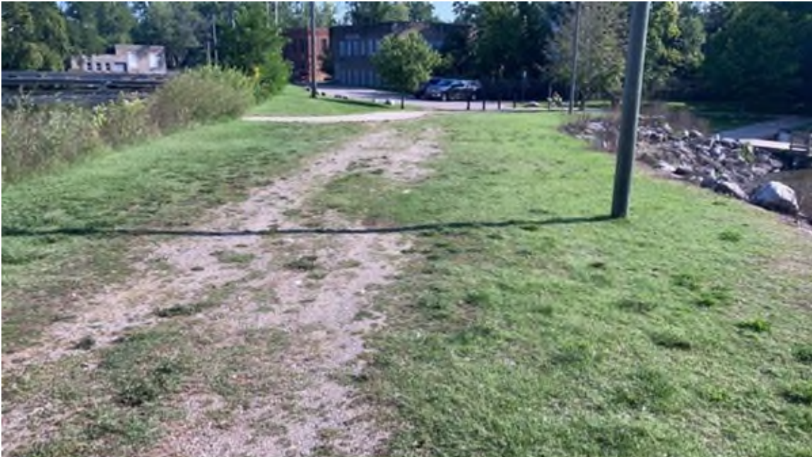
Photo #23 - Crest of left embankment. Note access trail on crest
