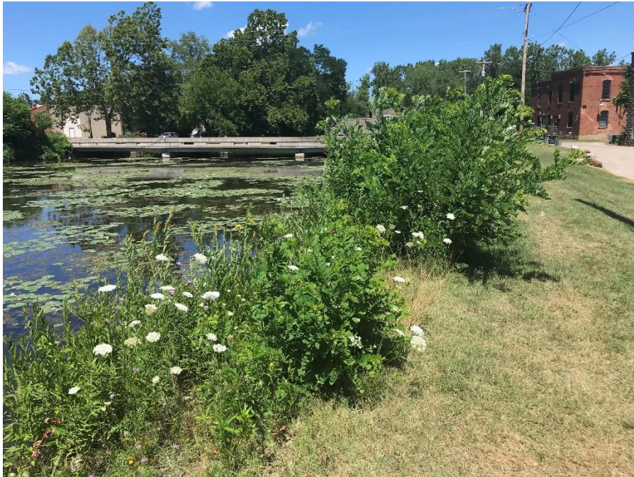
Photograph 7 – Upstream face of millrace embankment viewed from right Note the tall weeds and brush near the waterline
