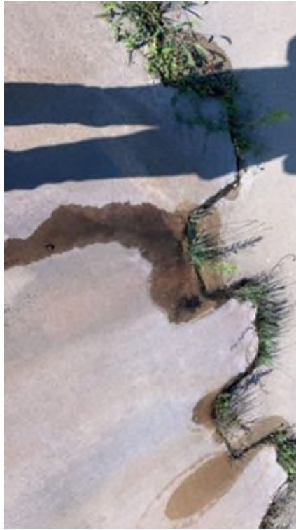
Photo #95 - Vegetation and water at sheetpile and concrete interface
