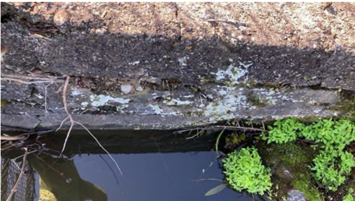
Photo #54 - Spillway right upstream abutment wall. Note concrete deterioration
