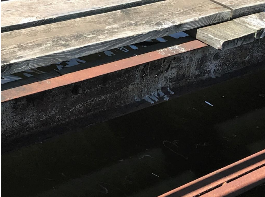
Photograph 24 – Deteriorated beam of catwalk
