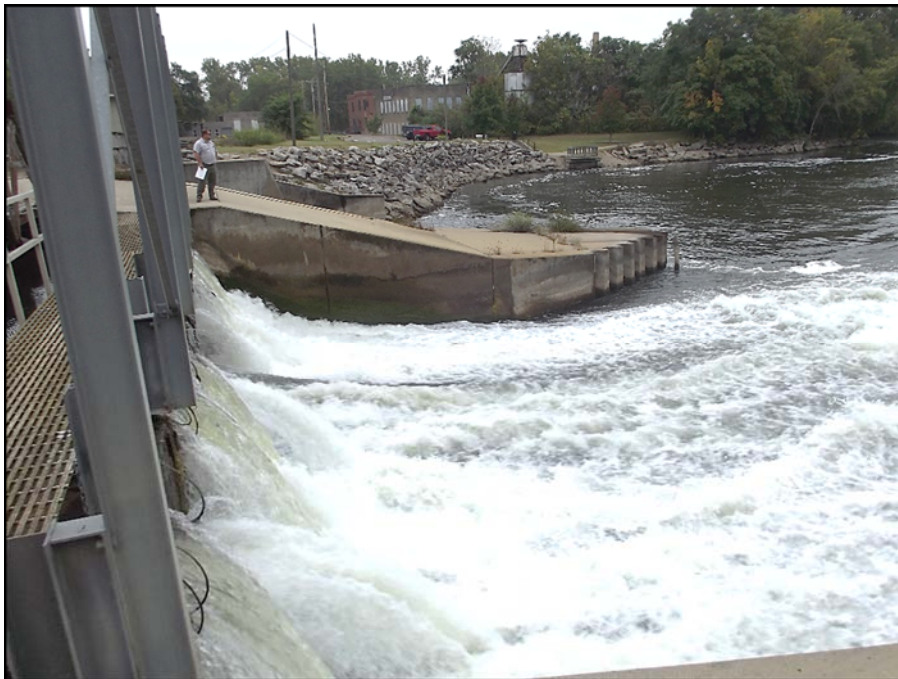
Photograph 20 – Needle section between Spillway Bays #2 and #3
