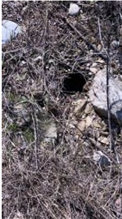
Photo #45 - Small animal burrow on left embankment
