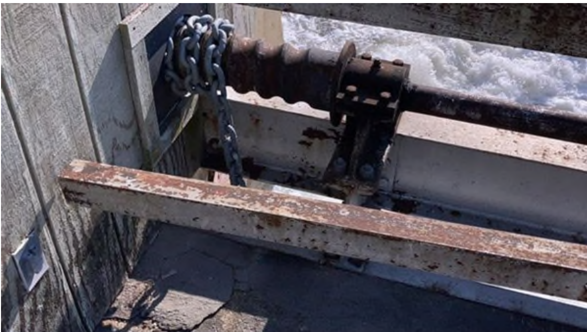
Photo #112 - Radial gate lifting chain and shaft
