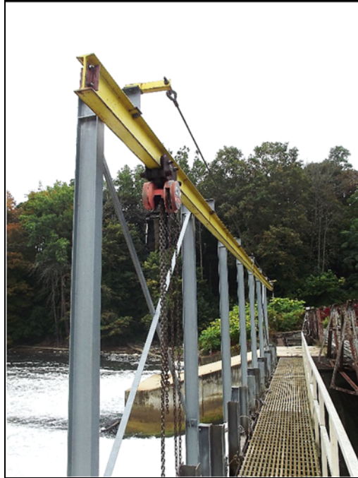
Photograph 17 – Spillway Bay #2 hoist system
