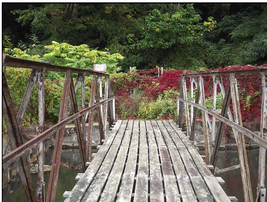
Photograph 8 – Right embankment crest viewed from left Note that deterioration of the catwalk prevents access
