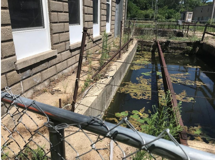
Photograph 26 – Concrete bulkhead at inlet to left section of powerhouse
