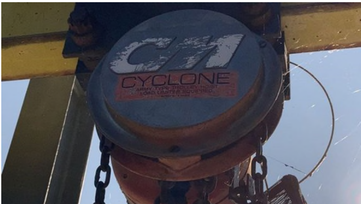
Photo #88 - Lifting mechanism for stoplogs of bay #2
