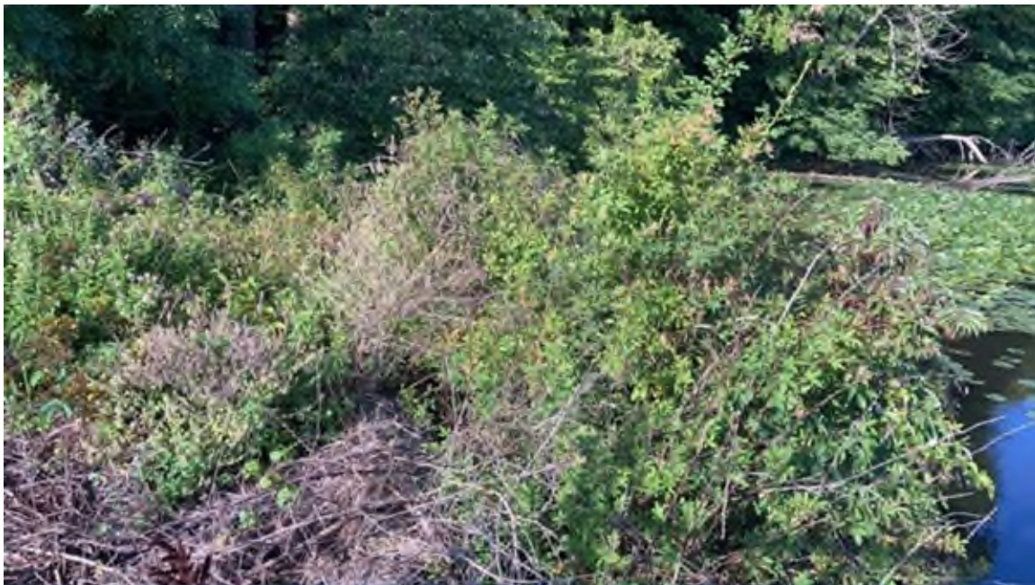
Photo #2 - Upstream slope right embankment, note brush growth
