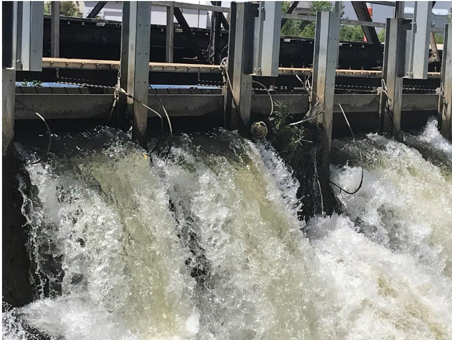
Photograph 21 – Stoplog and hoist cables viewed from downstream Note the significant leakage between stoplogs
