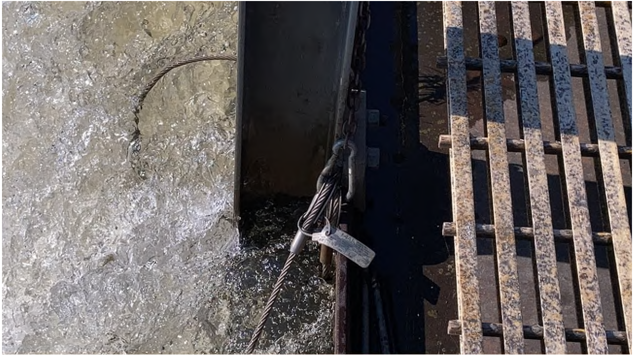
Photo #91 - Lifting cables on spillway bay #2 stoplogs
