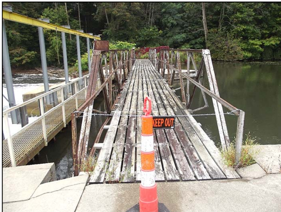
Photograph 18 – Catwalk over Spillway Bays #1 and #2 Note access has been prevented due to deterioration of the structure
