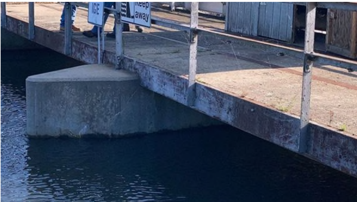
Photo #108 - Upstream pier between radial gate bays
