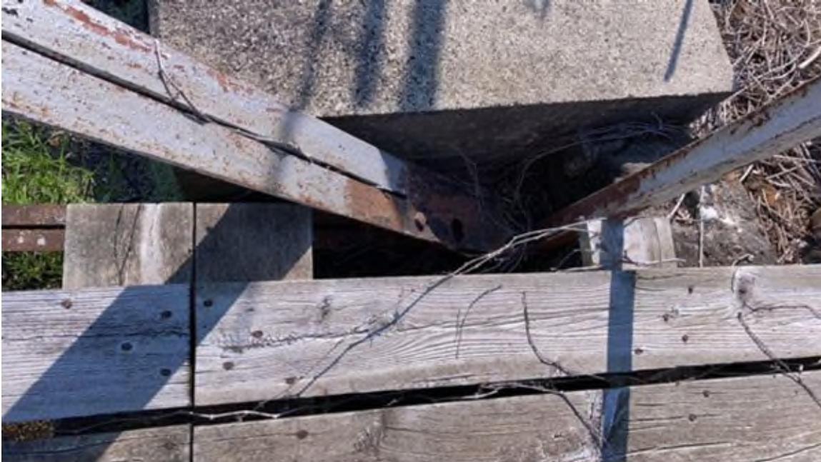
Photo #131 - Right end of walkway deck over spillway bay #1. Note this truss joint area is lower than the abutment walls, and water would overtop here first
