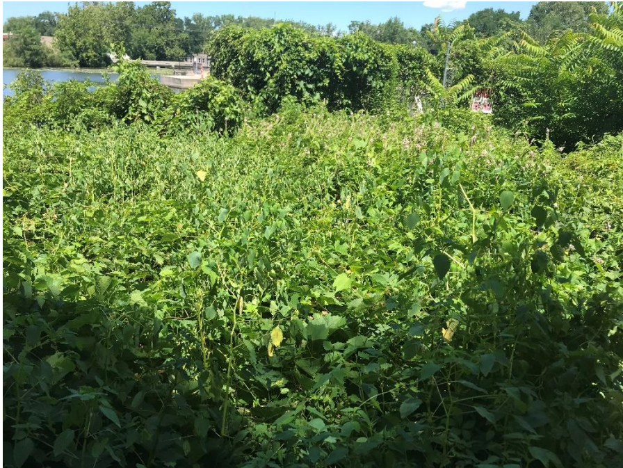
Photograph 5 – Right embankment crest viewed from right Note the tall weeds, brush, and small trees
