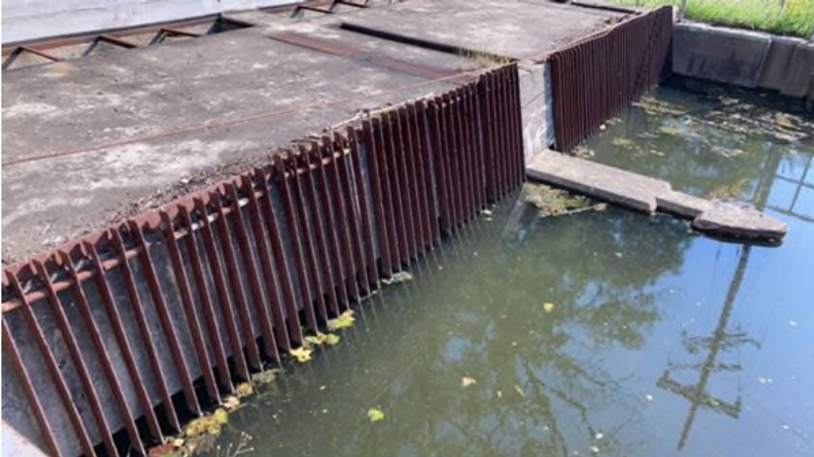
Photo #143 - Right side of powerhouse, inlet. No bulkhead exists
