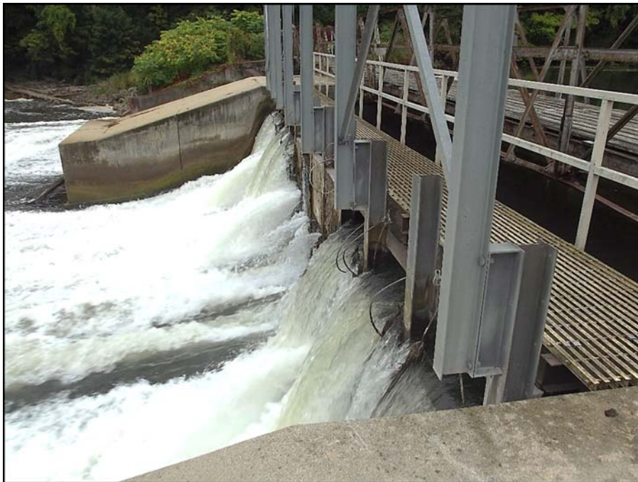
Photograph 16 – Spillway Bay #2, stoplog crests
