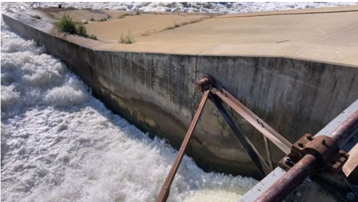
Photo #110 - Spillway bay #3 right downstream abutment and right gate pin
