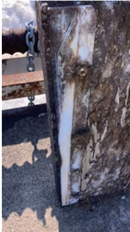
Photo #93 - Teflon strip along edge of spillway bay #2 stoplogs
