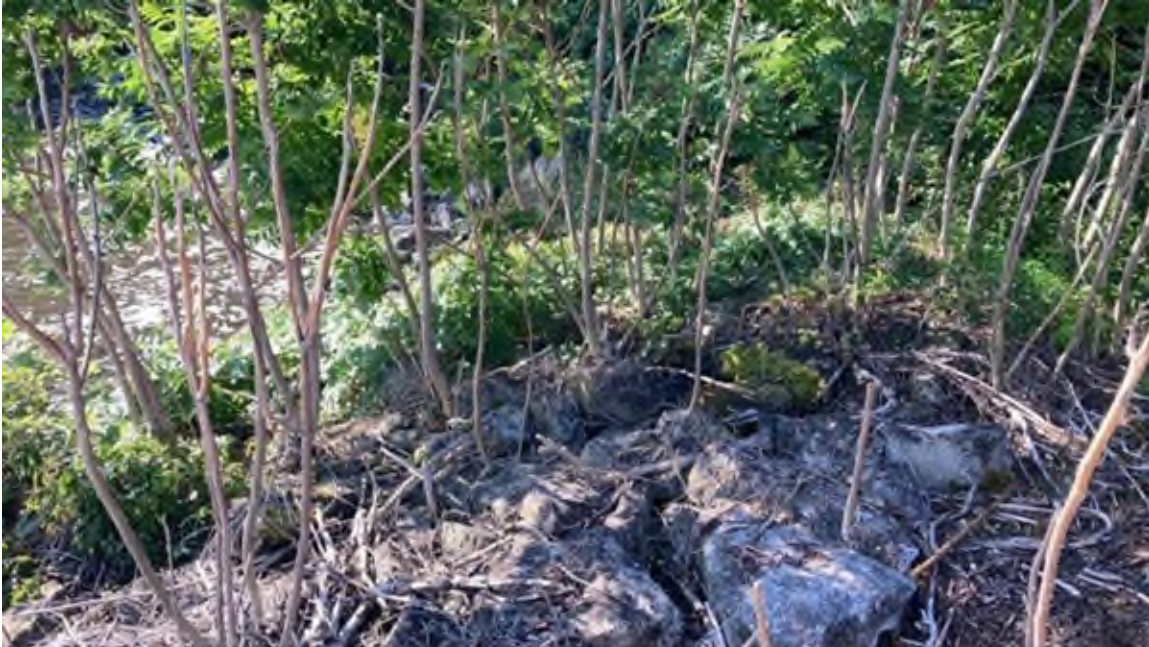
Photo #31 - Downstream slope of right embankment. Note brush growth within armoring
