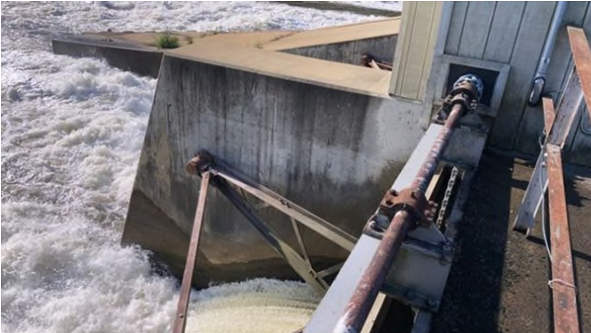
Photo #119 - Spillway bay #4 right downstream abutment wall and gate shaft
