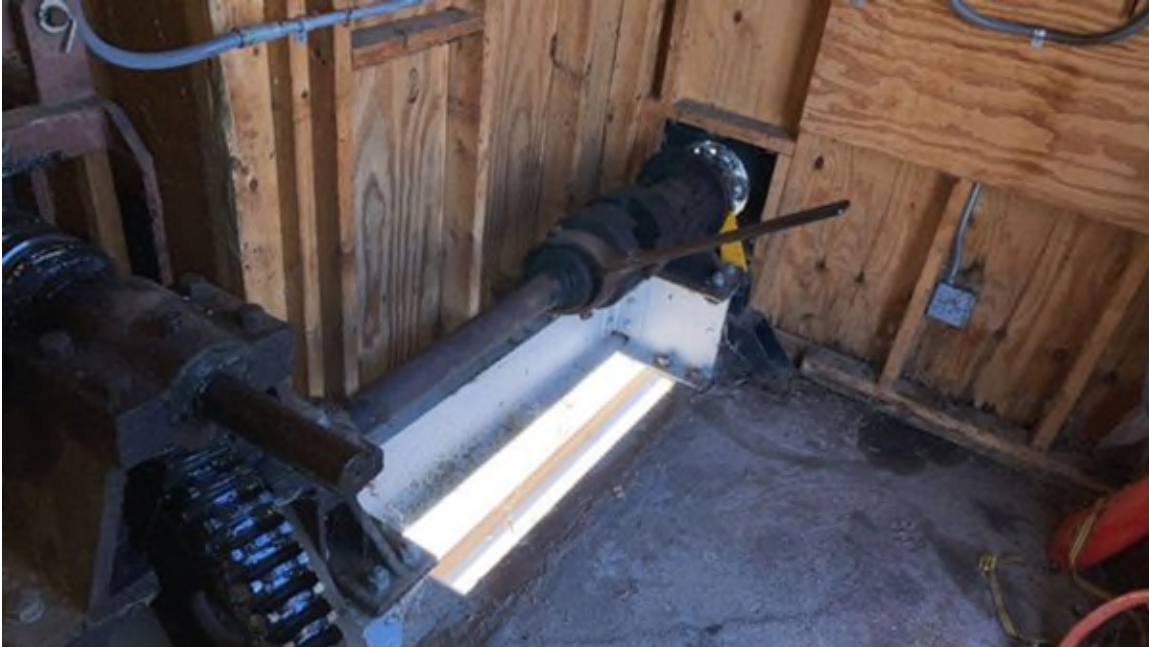
Photo #115 - Radial gate lifting shaft
