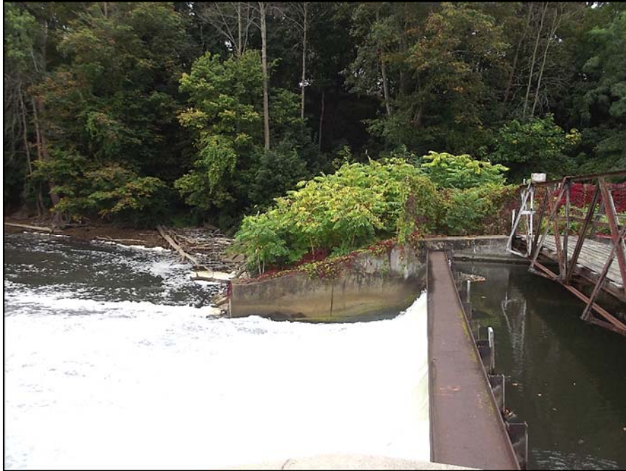
Photograph 9 – Downstream face of right embankment viewed from left Note that deterioration of the catwalk prevents access
