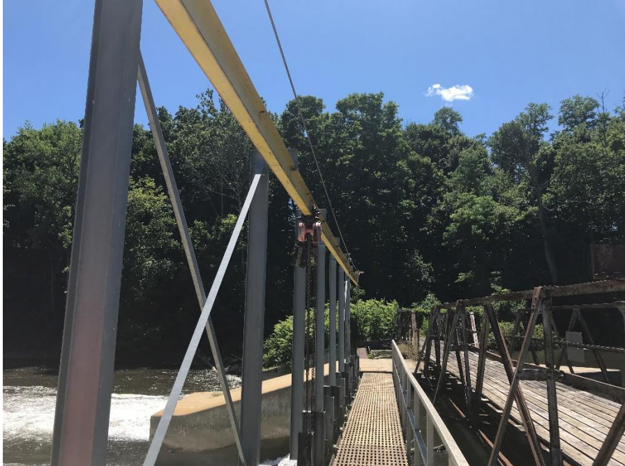
Photograph 20 – Catwalk and stoplog hoist system of center spillway
