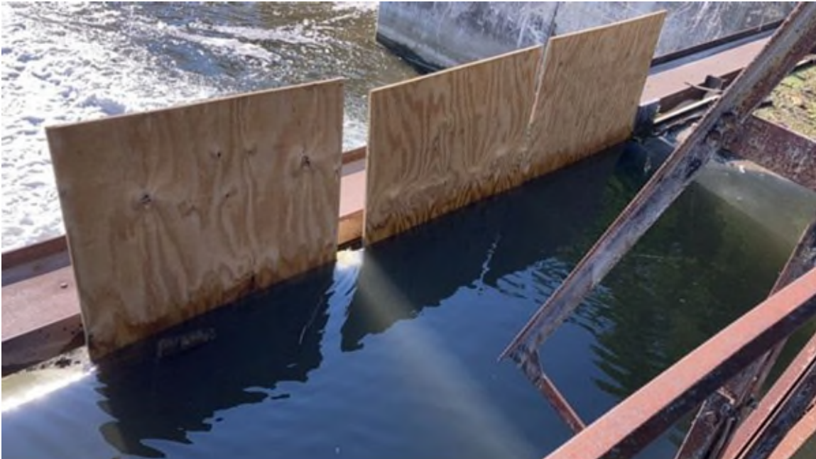
Photo #67 - Plywood placed upstream of some leaking stoplogs in spillway bay #1
