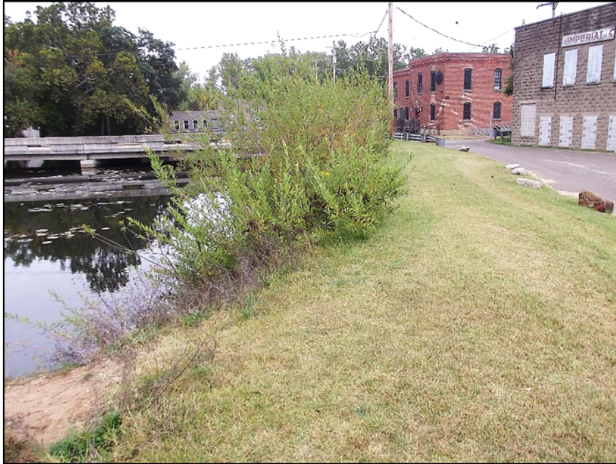
Photograph 1 – Upstream face of left embankment viewed from right Note the brush along the waterline
