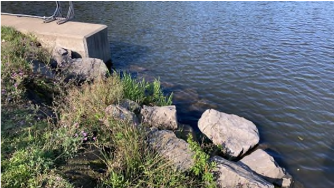
Photo #10 - Right end of left embankment upstream slope. Note riprap armoring
