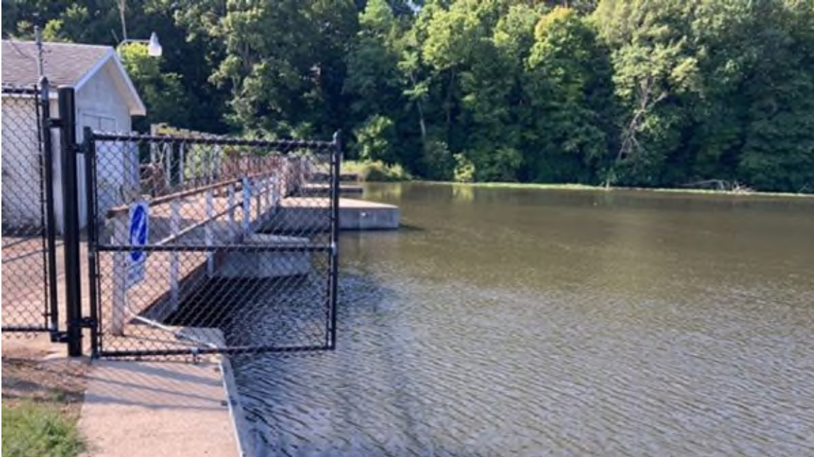
Photo #135 - Principal spillway inlet
