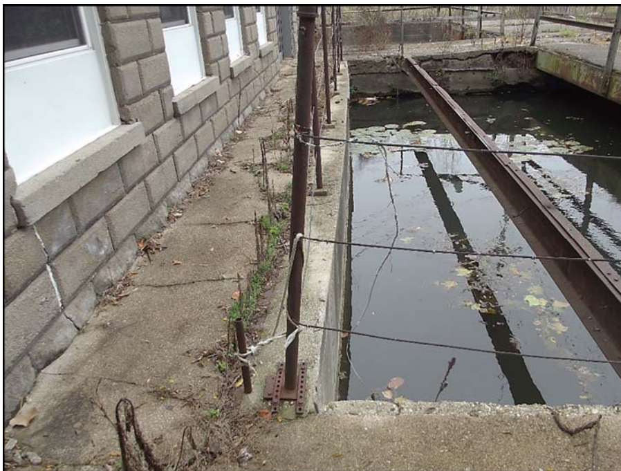
Photograph 26 – Concrete bulkhead at inlet to west section of powerhouse
