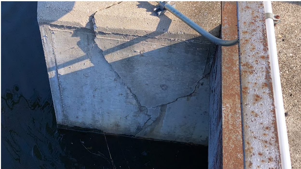
Photo #118 - Cracking on spillway bay #4 left upstream abutment
