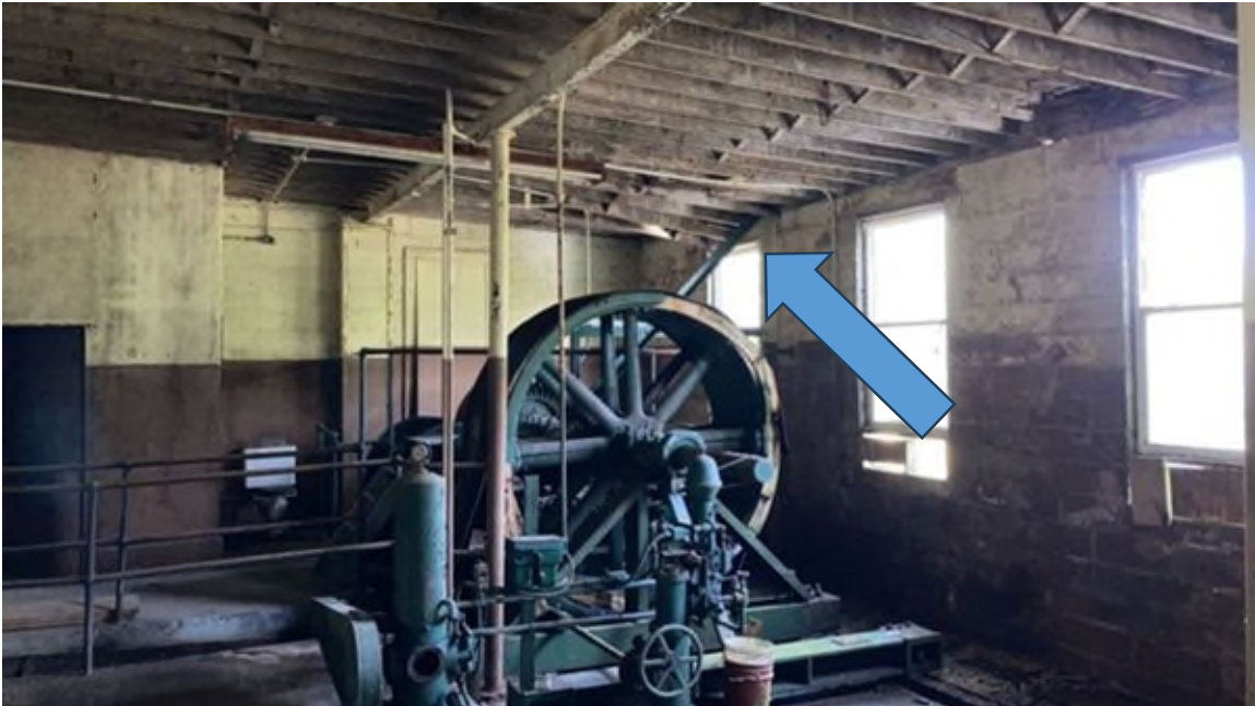
Photo #157 - Failing ceiling on left side of powerhouse
