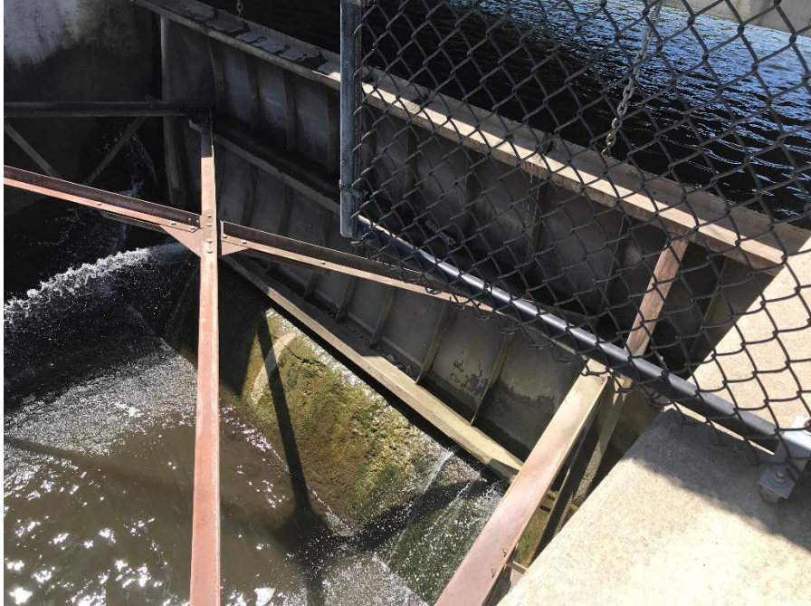
Photograph 16 – Typical radial gate viewed from downstream
