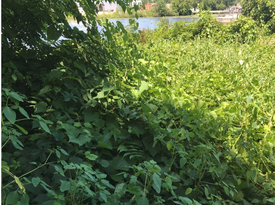
Photograph 4 – Upstream face of right embankment viewed from right Note the tall weeds, brush, and small trees
