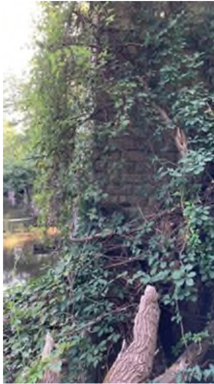
Photo #161 - Powerhouse left face. Note significant vegetation growth up wall
