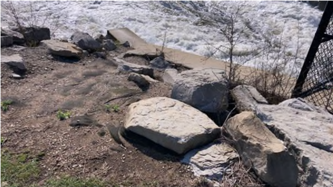
Photo #39 - Downstream slope of left embankment adjacent to spillway. Note exposed fabric where armoring is missing
