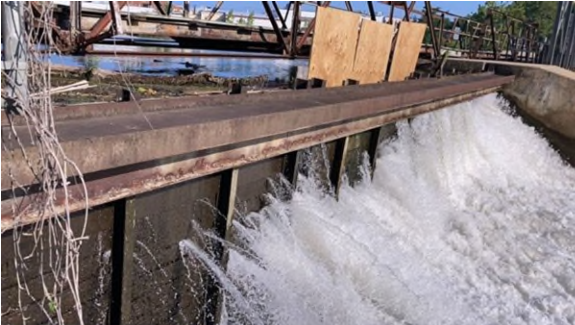
Photo #63 - Spillway bay #1. Beam at top of stoplog grooves appears slightly sagged
