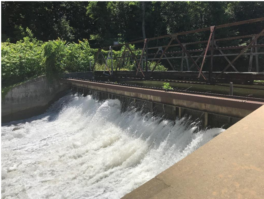
Photograph 22 – Right stoplog spillway viewed from downstream
