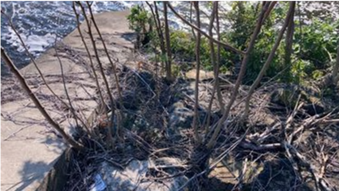
Photo #30 - Downstream slope of right embankment adjacent to spillway. Note brush growth
