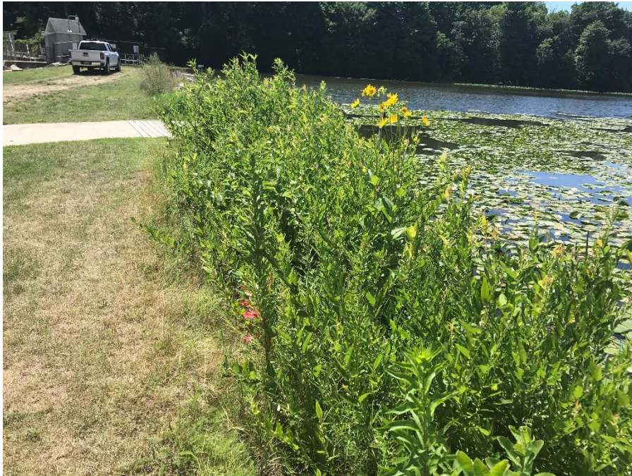
Photograph 1 – Upstream face of left embankment viewed from left Note the tall weeds along the waterline
