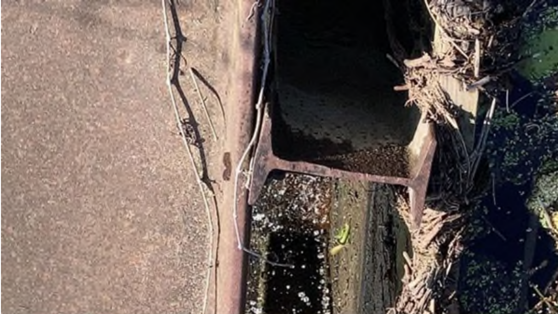
Photo #75 - Stoplog groove for spillway bay #1
