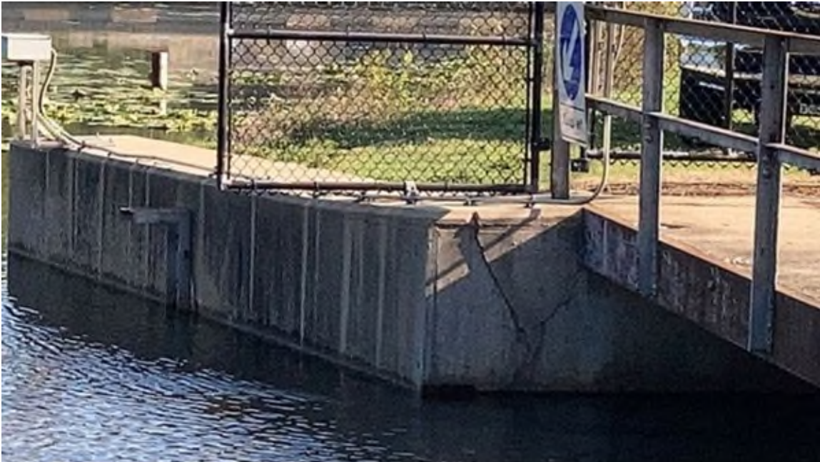
Photo #109 - Spillway bay #4 left upstream abutment. Note cracking
