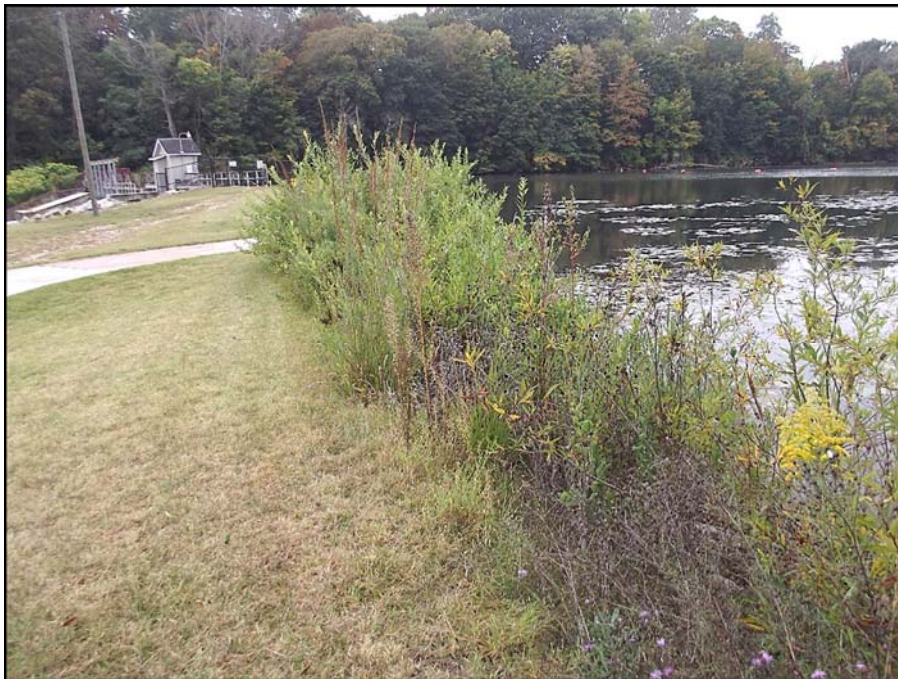
Photograph 4 – Upstream face of left embankment viewed from left Note brush along the waterline
