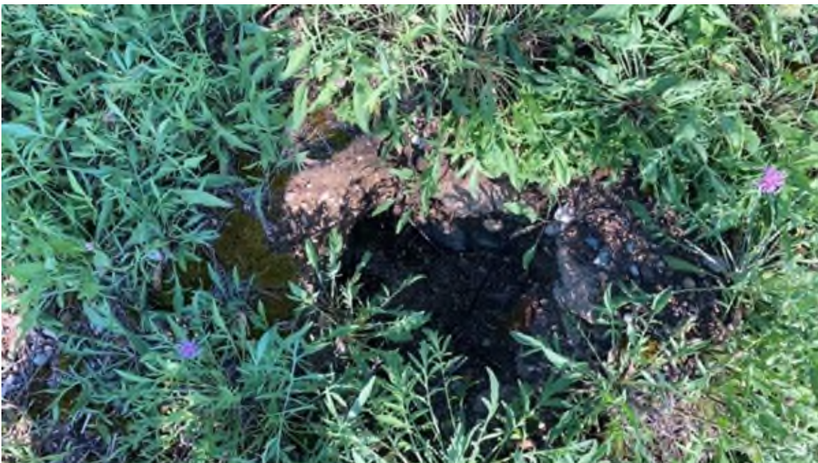
Photo #52 - Burrow or sinkhole on left embankment adjacent to millrace
