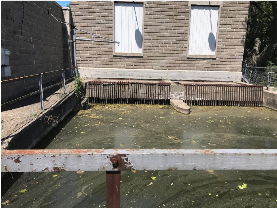
Photograph 27 – Gated inlet to right section of powerhouse
