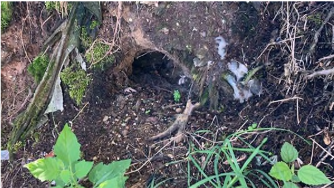
Photo #50 - Burrow on embankment near powerhouse outlet
