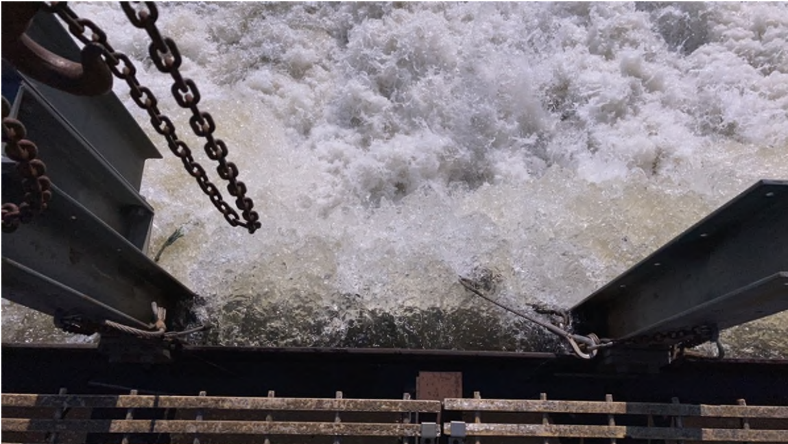
Photo #89 - Individual stoplog bay of spillway bay #2. Bays consist of three logs on top of one another that can all be removed
