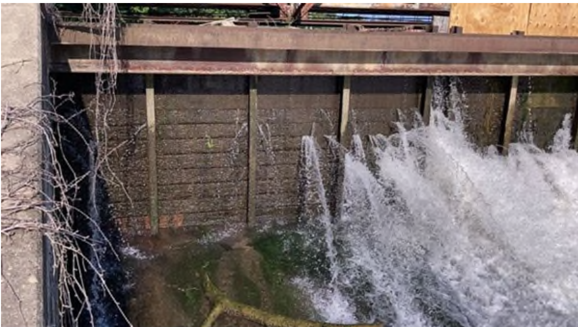
Photo #60 - Wooden stoplogs of bay #1, significant leakage observed
