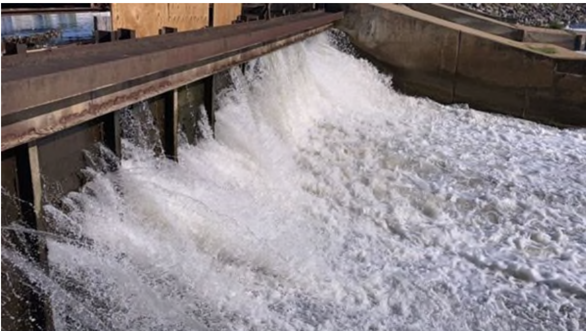
Photo #62 - Wooden stoplogs of bay #1, significant leakage observed
