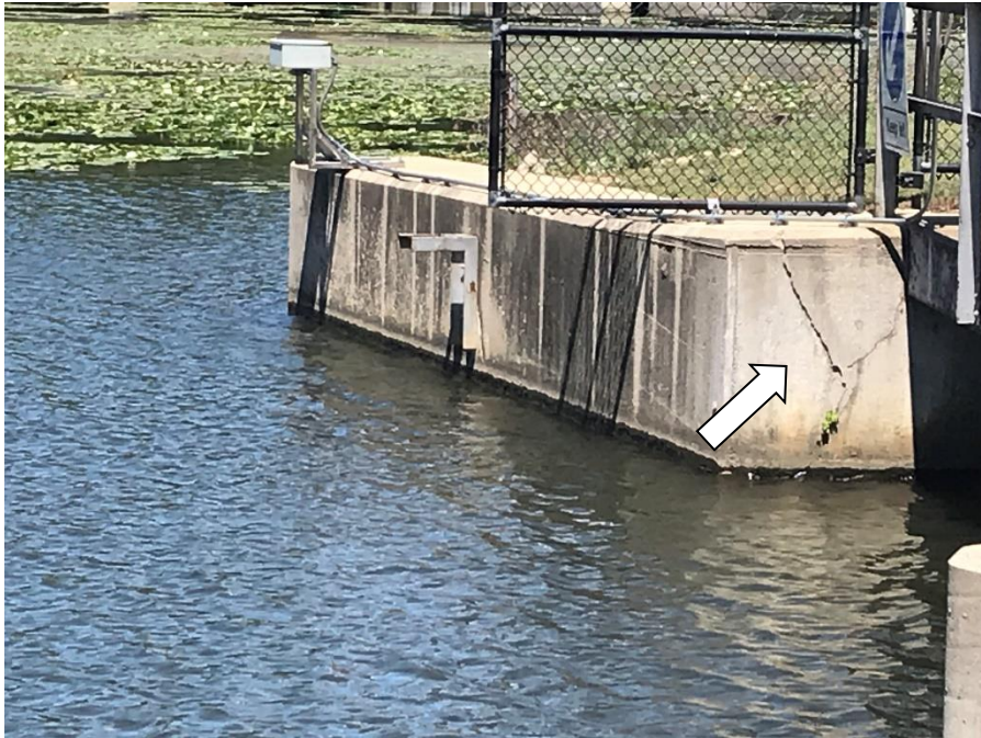
Photograph 11 – Upstream left abutment wall Note the cracks near the catwalk connection
