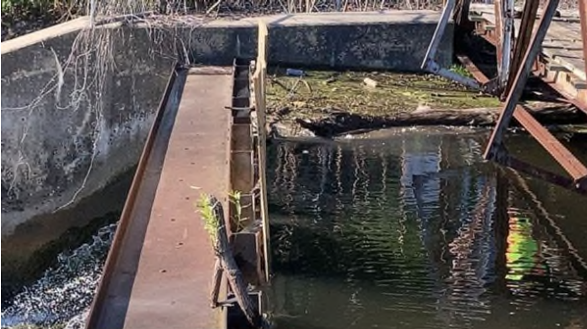
Photo #73 - Spillway bay #1, minor deflection downstream
