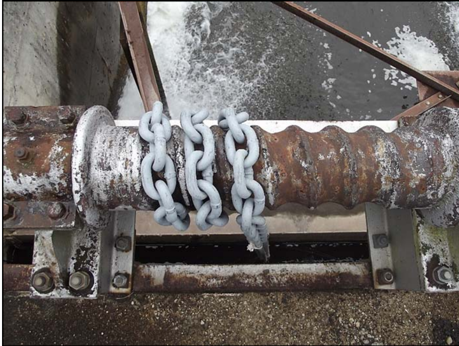
Photograph 23 – Typical radial gate hoist chain
