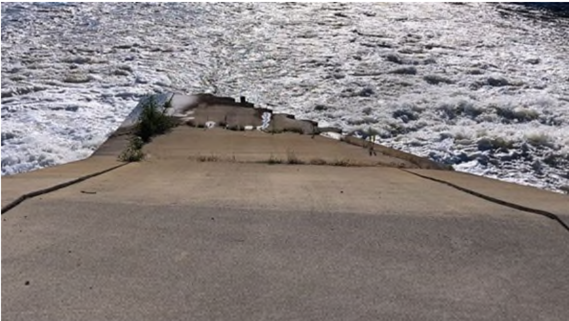
Photo #84 - Downstream needle section of abutment between spillway bays #2 and #3
