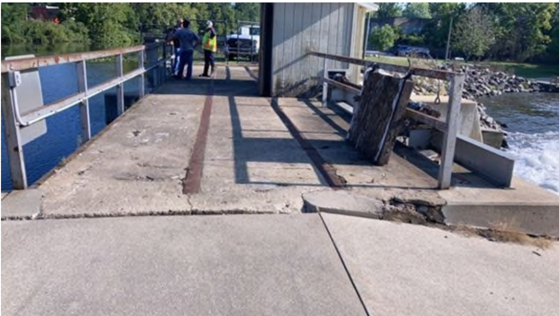
Photo #106 - Deck over spillway bays #3 and #4. Note deteriorating concrete on downstream (right in photo) side of deck at joint with abutment
