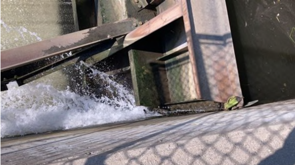
Photo #123 - Leakage at left edge of spillway bay #4 gate
