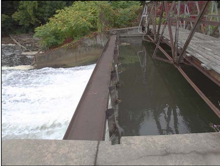
Photograph 15 – Spillway Bay #1, stoplog crests
