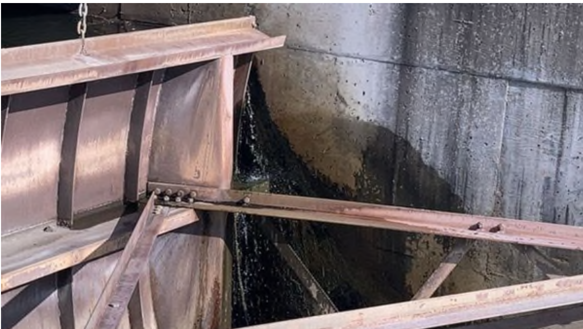
Photo #102 - Minor leakage along left side of spillway bay #3
