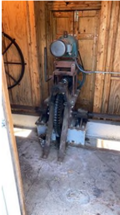
Photo #113 - Radial gate lifting motor
