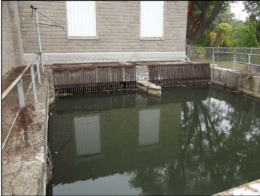
Photograph 27 – Gated inlet to east section of powerhouse
