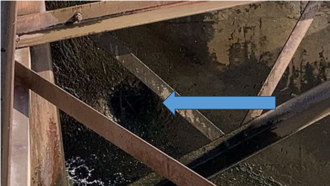
Photo #103 - Hole in left wall of spillway bay #3
