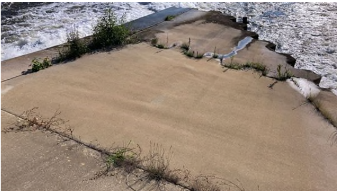
Photo #94 - Downstream needle section between spillway bays #2 and #3. Note some vegetation growing within joints and sheetpile interface with water seeping down
