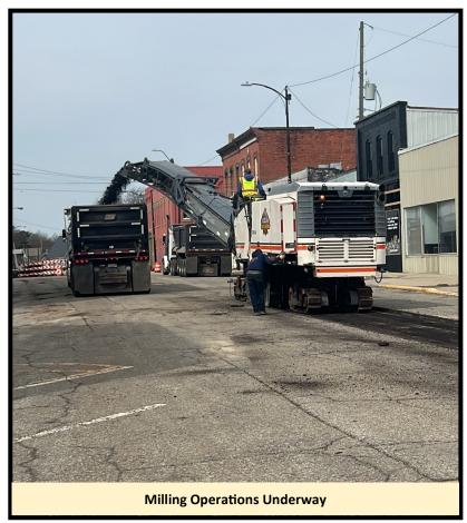
Milling the pavement allows for the asphalt material to be easily separated from the bricks below, and be recycled for use in future asphalt paving projects. After the roadway surface is milled, excavators are put to use removing the underlying bricks and concrete pavement that existed underneath the asphalt.
