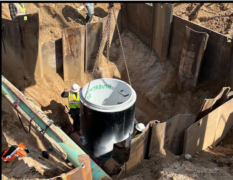
Placing new manhole on existing sewer to connect to the new sewer
