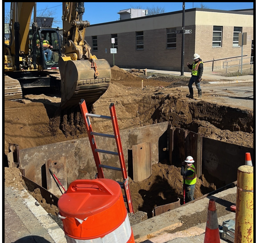
Sanitary Sewer Installation Underway
