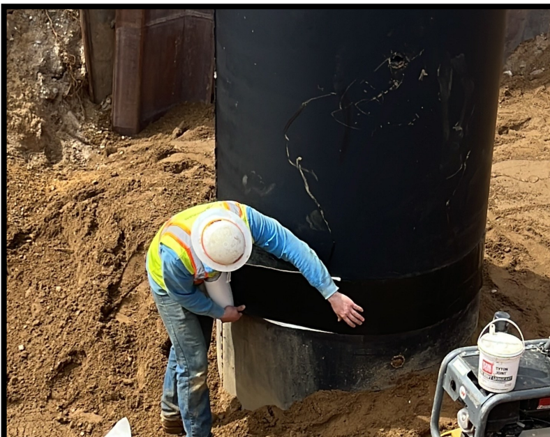
A new manhole is placed along the new sanitary line and backfilled
