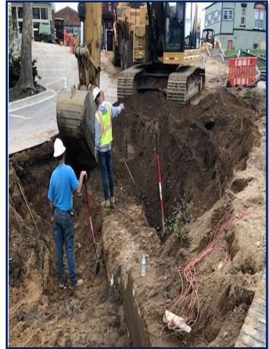
Fig 1: Encountering a masonry wall underneath the road
