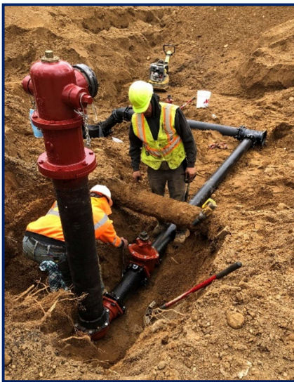
Fig 2: New fire hydrant installation along Brady St.
