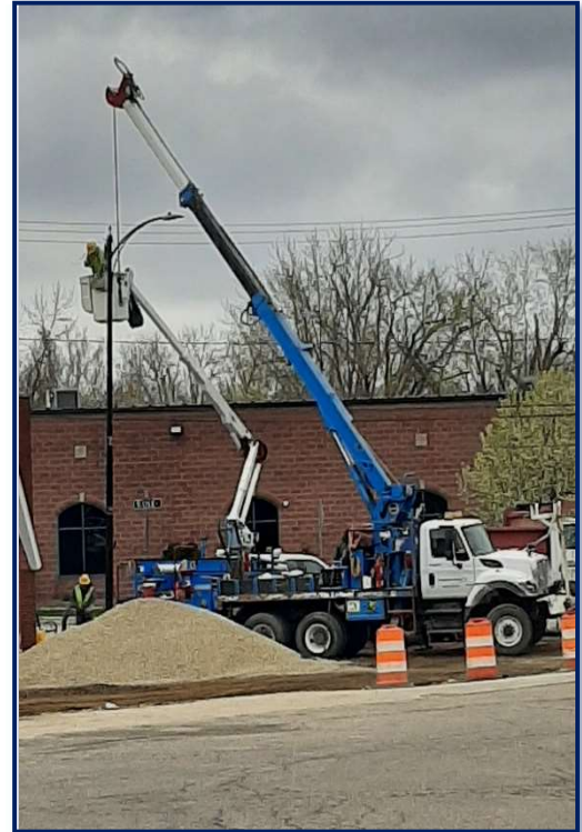
Fig 1: Consumers Energy removing light poles to prepare for replacements.
