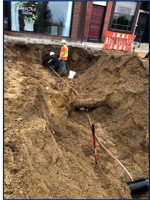
Fig 1: Milbocker installing new water services on Brady St.
