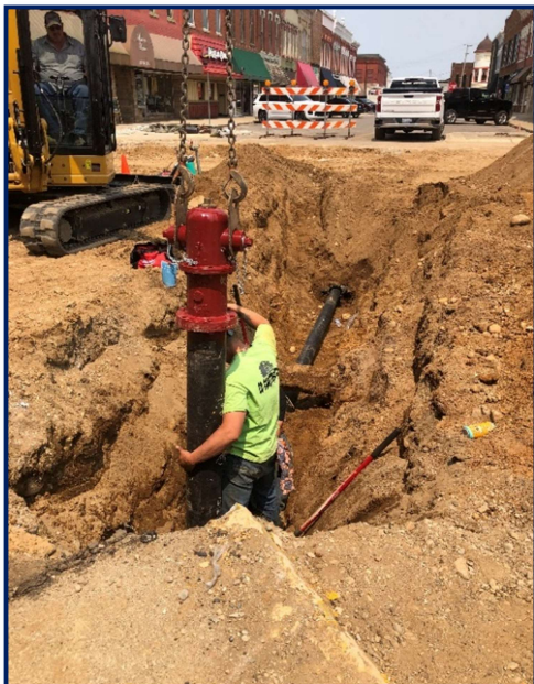
Fig 2: Milbocker installing a new fire hydrant on Hubbard Street
