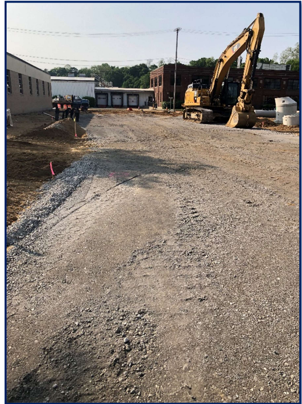
Fig 1: Road grading along Brady St. has been completed up to aggregate base
