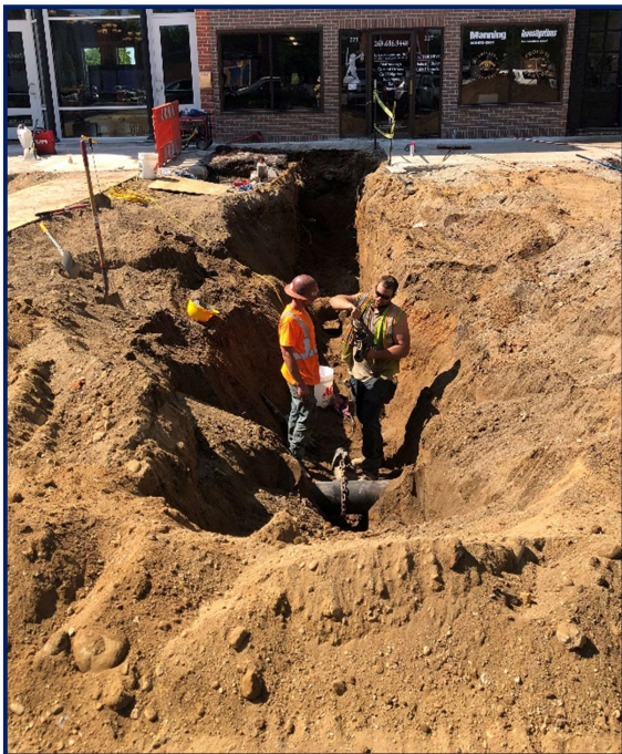
Fig 2: Milbocker continues to install water services to residents of downtown Allegan.
