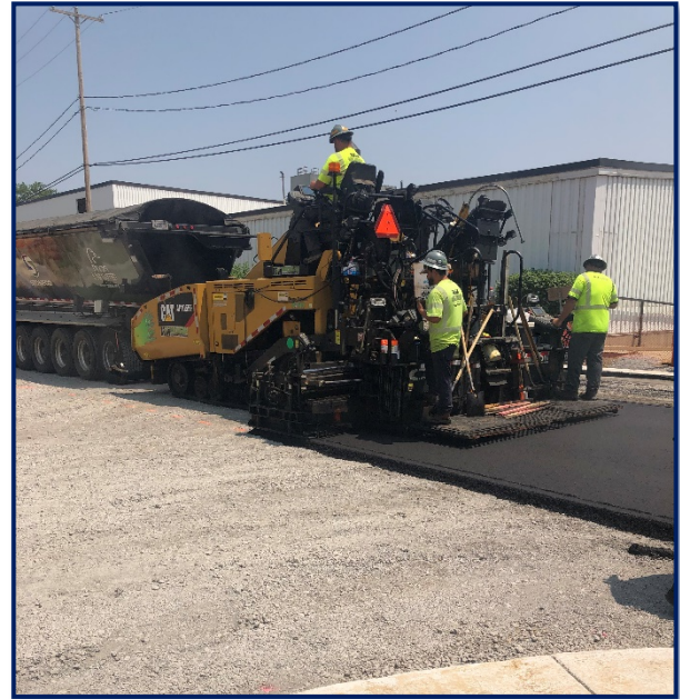
Fig 1: Michigan Paving lays asphalt on State Street
