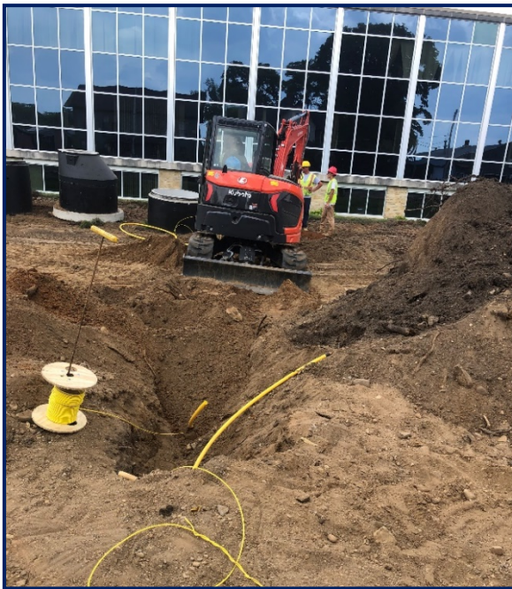
Fig 2: Michigan Gas replaces gas services along Riverfront Plaza
