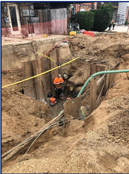
Fig 2: Existing seawall from 1947 found on Riverfront Plaza
