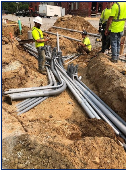
Fig 2: Severance prepares conduit sweeps for electrical handholes
