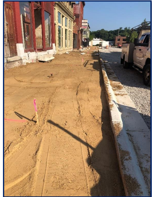
Fig 1: Milbocker continues sidewalk removals along Brady Street
