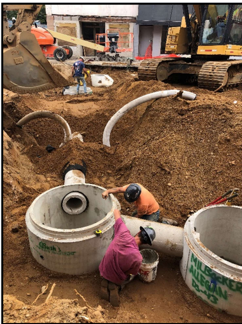
Fig 2: Milbocker crews continue storm sewer installation on Locust St.
