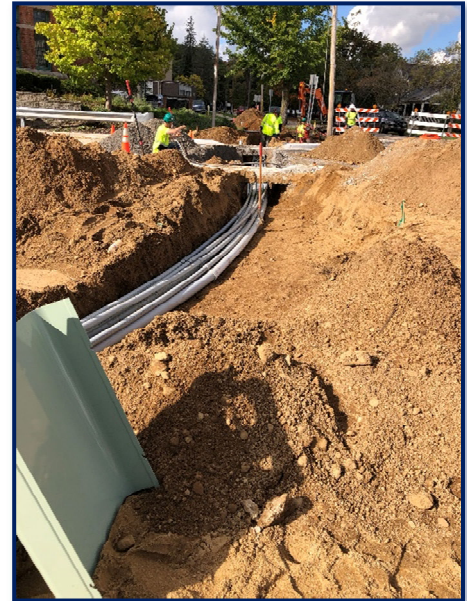
Figure 1: Conduit continues to be installed by Severance Electric along Hubbard Street.
