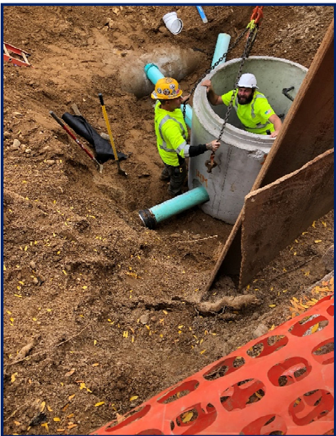
Figure 2: Milbocker installs another stormwater catch basin on Trowbridge Street.
