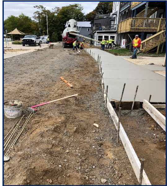
Figure 1: Crews from Duran Concrete pour sidewalks along Riverfront Plaza.
