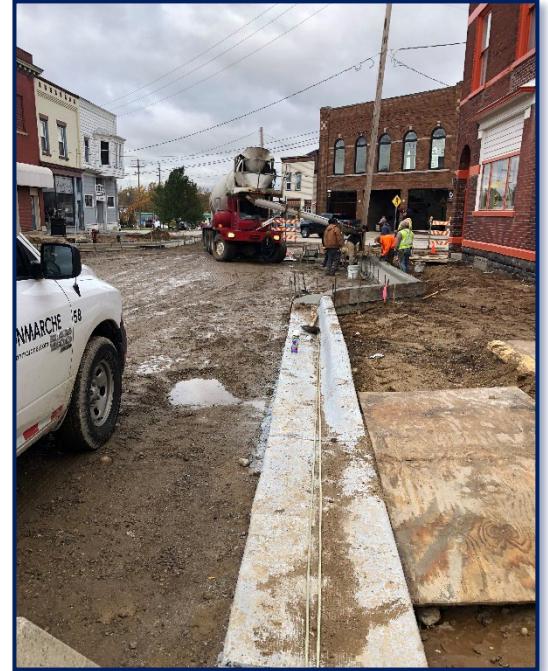
Figure 1: Crews from Duran Concrete install curb and gutter along Locust Street.
