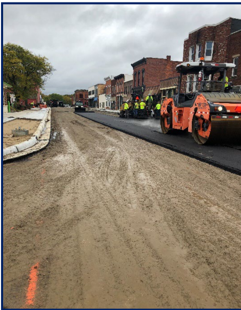
Figure 2: Michigan Paving laying a base layer of asphalt on Hubbard Street.
