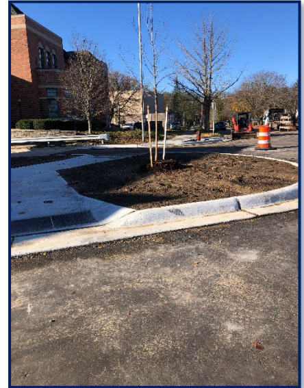
Figure 1: Newly installed planting area near intersection of Hubbard and Walnut.
