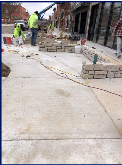
Figure 2: Seat wall and pedestrian area taking shape.
