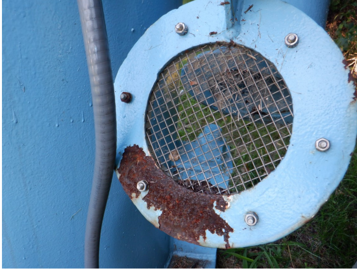
16) The screen is in good condition but is oversized.
