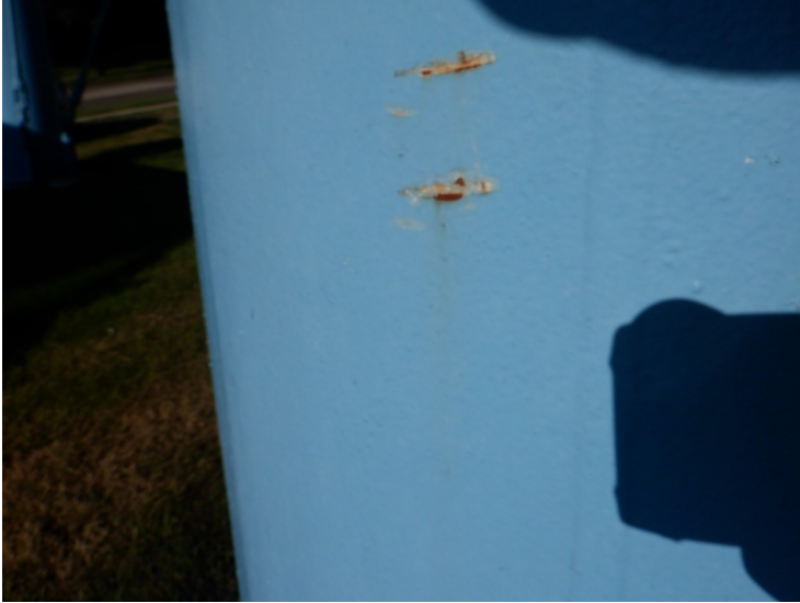
22) Spot failures on the legs.
