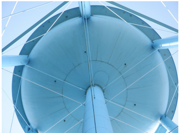
26) The coating on the bowl is in good condition.
