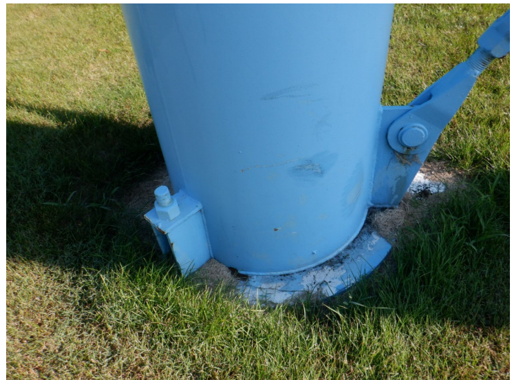
11) There is soil covering some of the leg foundations.
