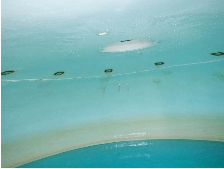
46) The coating on the roof is in good condition overall.
