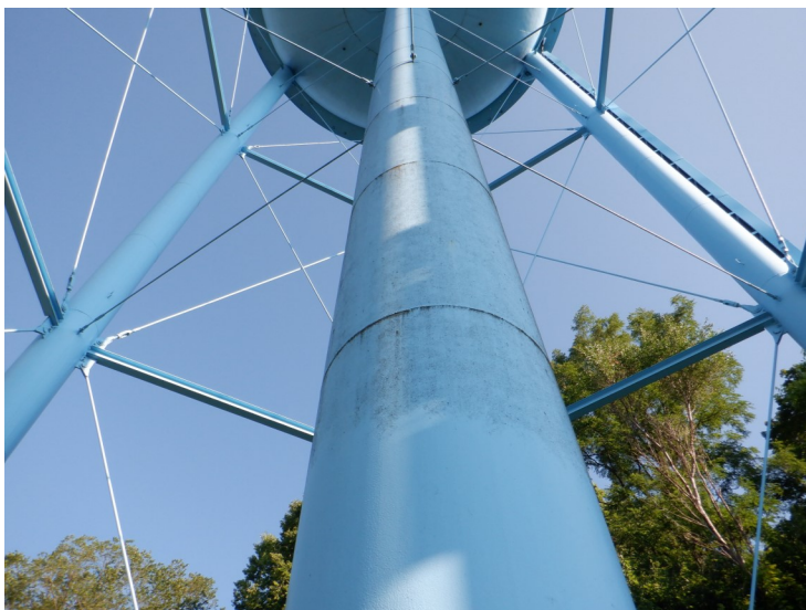
6) The coating on the riser is in good condition overall.
