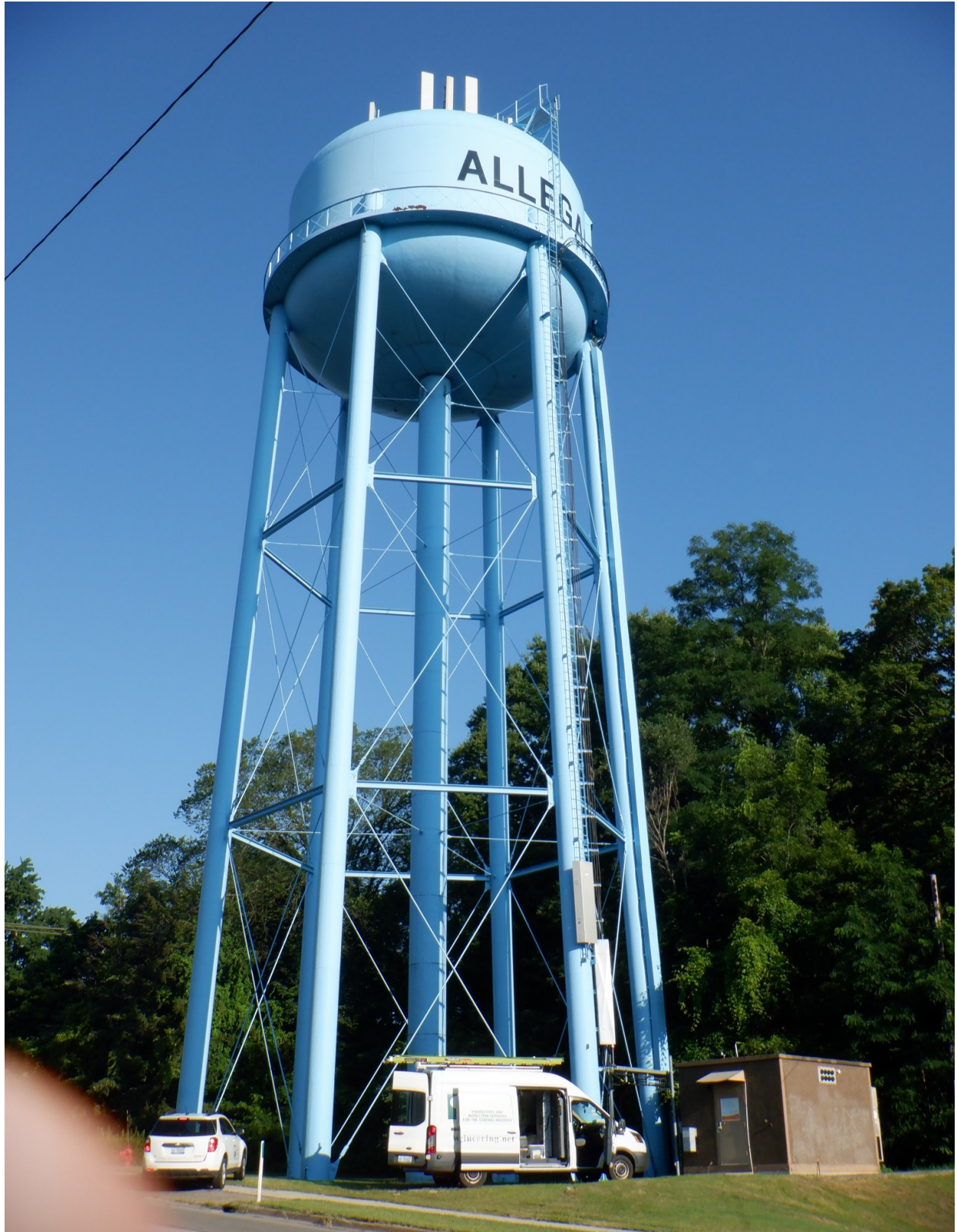
250,000 gallon double ellipse (West) elevated water storage tank located in Allegan, Michigan.
