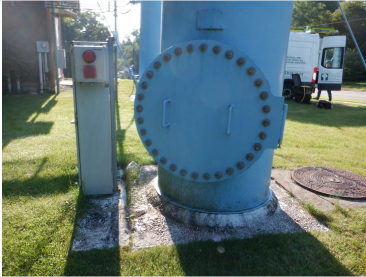
4) The riser manway is in good condition.
