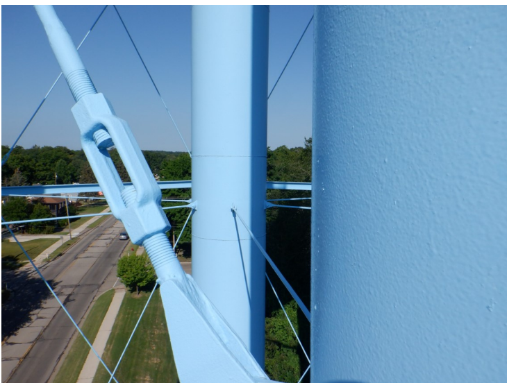
24) The sway rods are in good condition.
