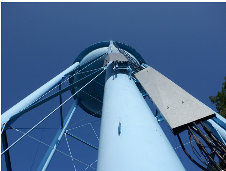
18) The leg ladder has a vandal guard.
