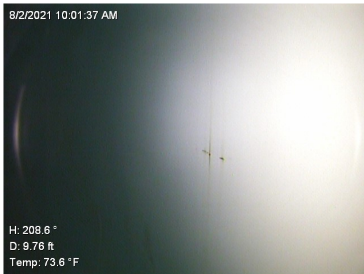
52) Spot coating failures on the sidewall.
