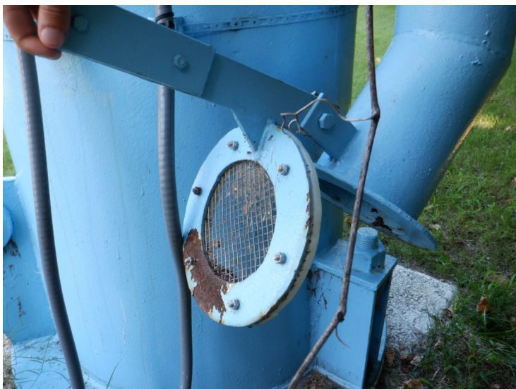
15) There is a screened flap gate at the discharge end of the overflow pipe that is in good condition.
