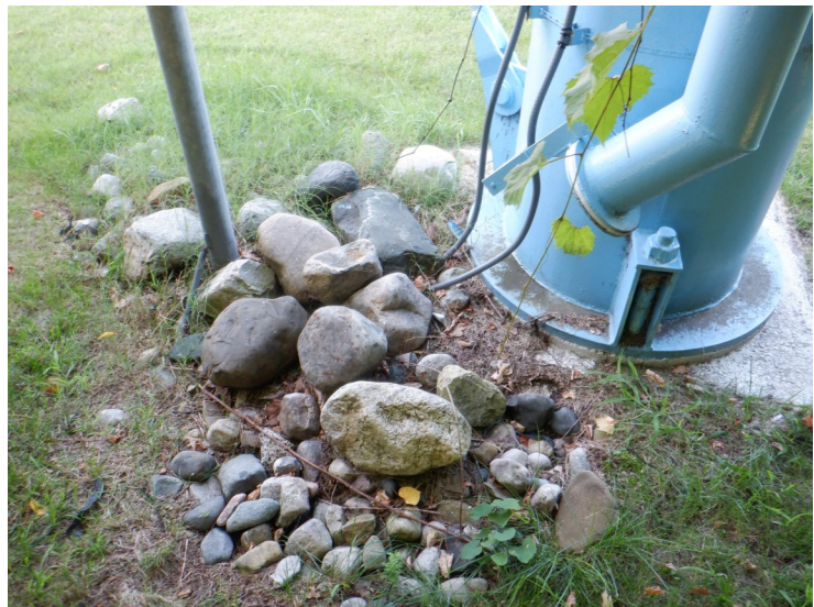
14) The overflow pipe is in good condition.
