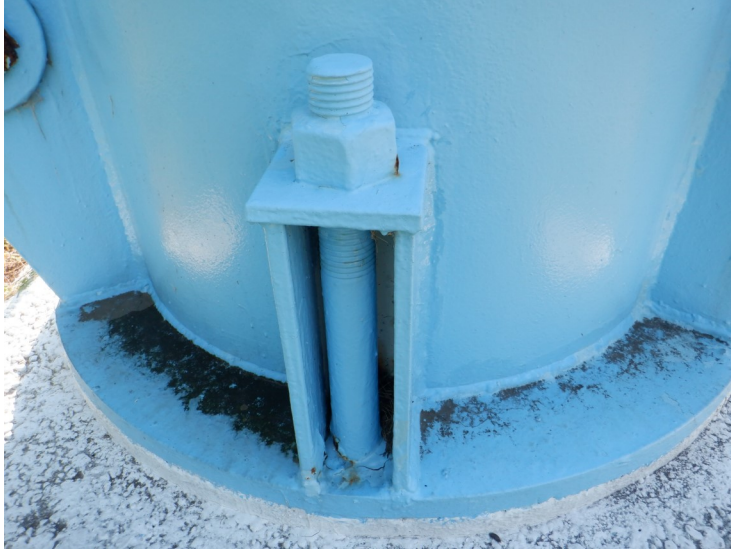
13) Typical leg anchor bolt is in good condition.
