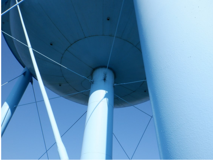
25) The riser rods are in good condition.
