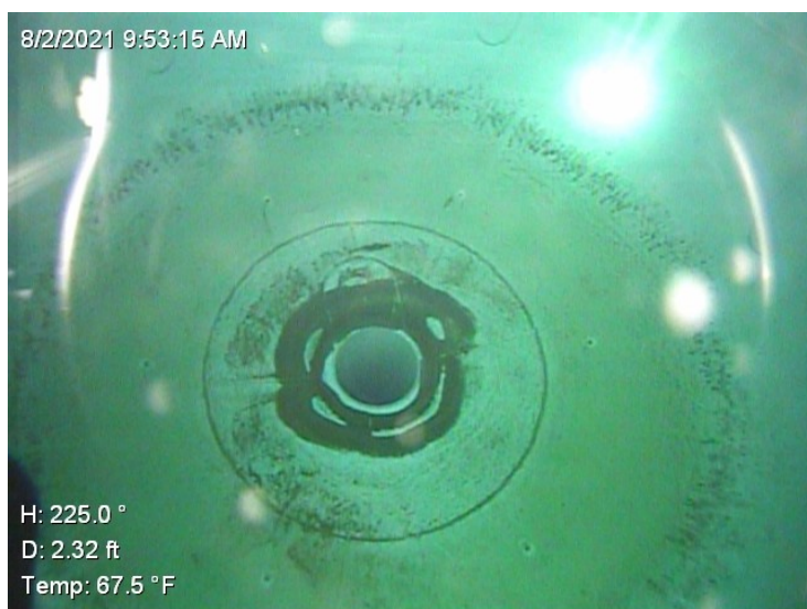
54) The coating on the bowl is in good condition.
