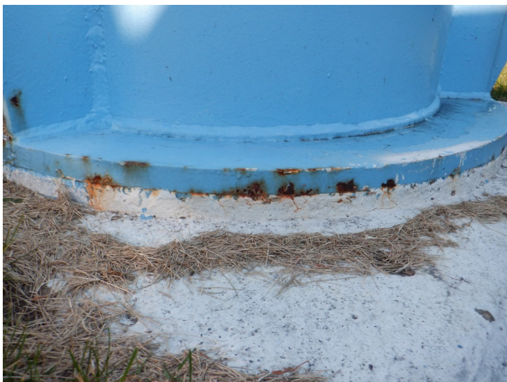
12) The leg grout is in good condition.
