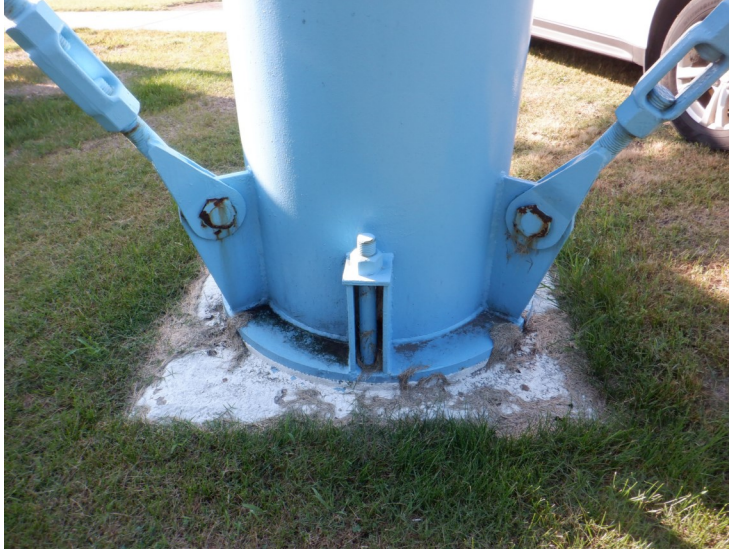
10) The leg foundation is in good condition.
