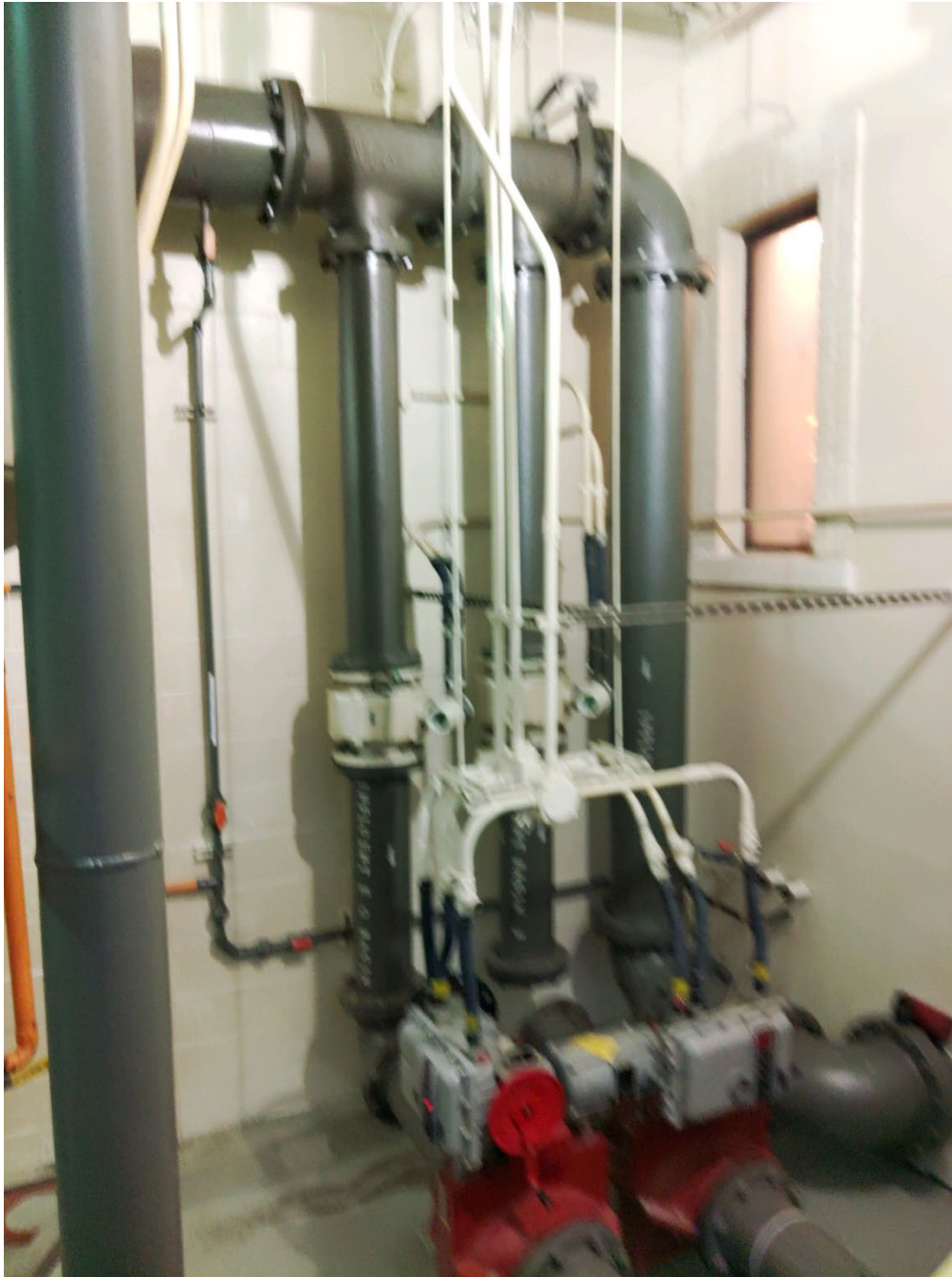
Diverting lines to EQ basin and basin 3
