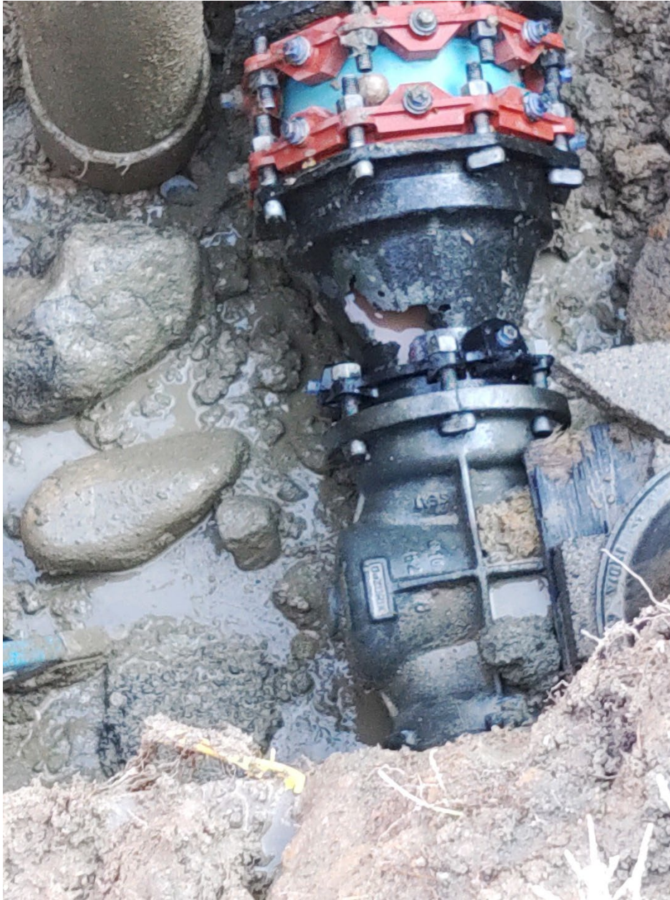
Damaged force main
