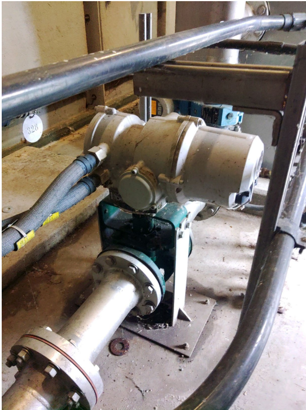
Rotork valve in septage
