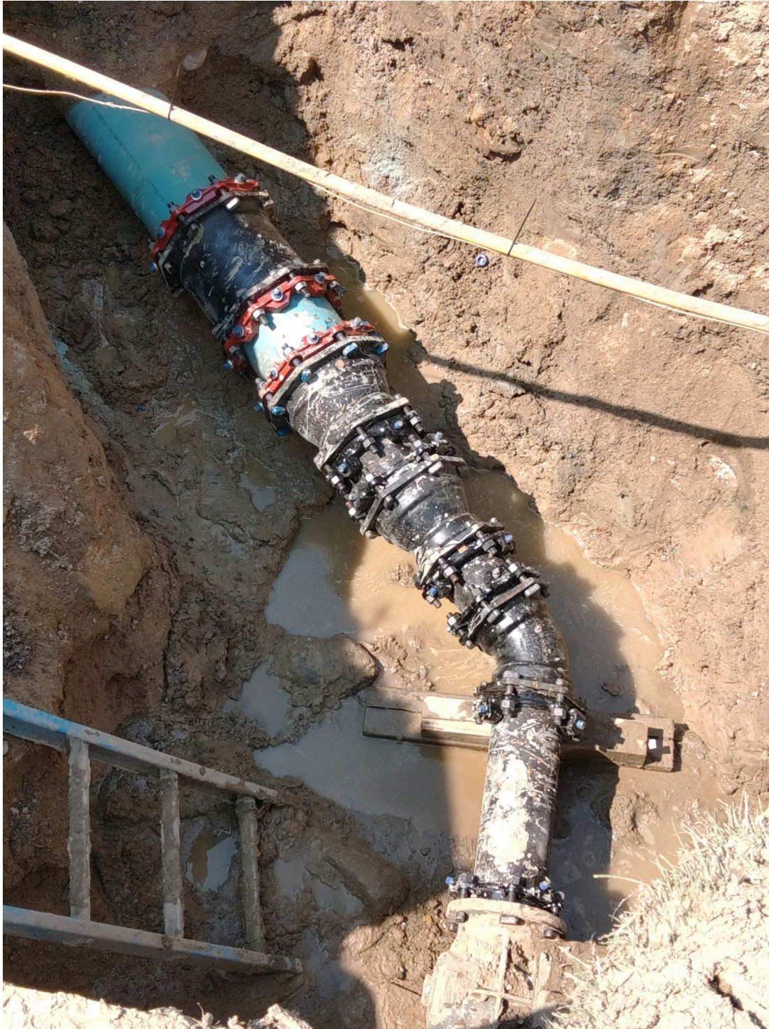
Emergency repaired force main
