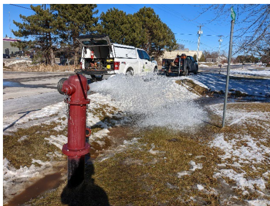
Hydrant flushing at the intersection of Paad Court and Michigan Avenue
