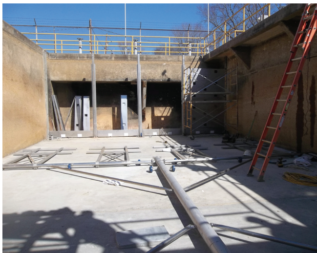
Dewberry assisted HCSA with a solids diversion project including installation of an automated sludge removal system.
