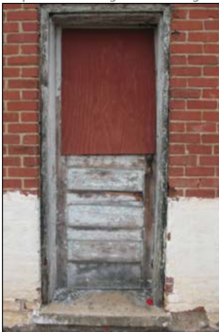
Figure 23- Wood doors are susceptible to moisture damage if not kept protected with paint. Here, broken glass is covered with plywood and the rails of the door exhibit significant damage. Also visible in this photo is a deteriorating lime wash on the base of the building.
