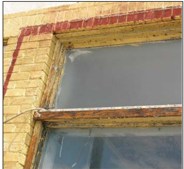
Figure 19- Broken glass and wood that is left unpainted are common maintenance problems for storefronts. Unpainted wood is not protected from weather.
