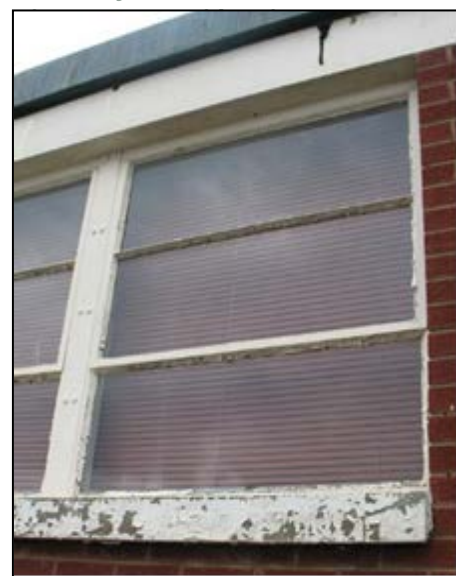
Figure 26- Metal windows are common in Altavista; typical maintenance problems include damaged glazing putty and deteriorating paint. Both can lead to rust and further problems including warping.
