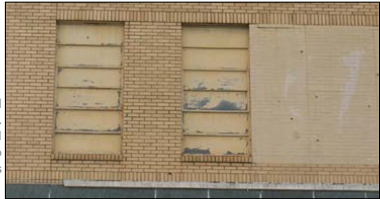
Figure 24- Window openings that have been filled with brick detract from the commercial district. Missing flashing between different materials and caulking between stone panels can lead to moisture problems
