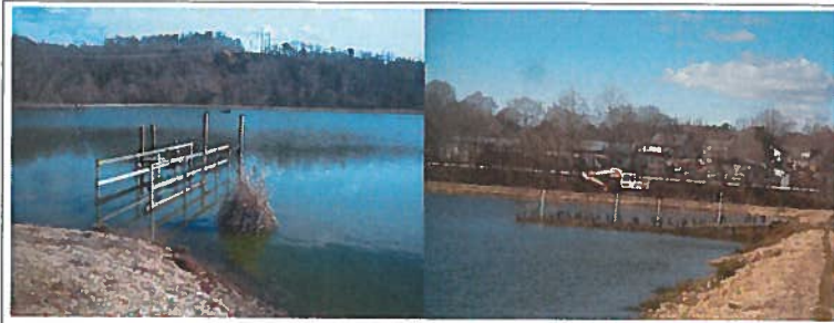
Figure 5-9: Wastewater overflow lagoon at Altavista. Some floating piers have been established for sediment sampling (left photo). Plot #7 established by Ecolotree Inc. to investigate the PCB degradation in a hot spot using hybrid poplar and willow trees deeply rooted throughout the contaminated zone (right photo). Images courtesy of Gabriele Ludewig, isrp.
