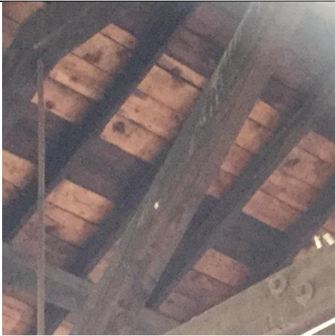
Roof – Wood planking
