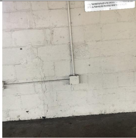
Interior Walls- masonry block, rough surface in fair to good condition
