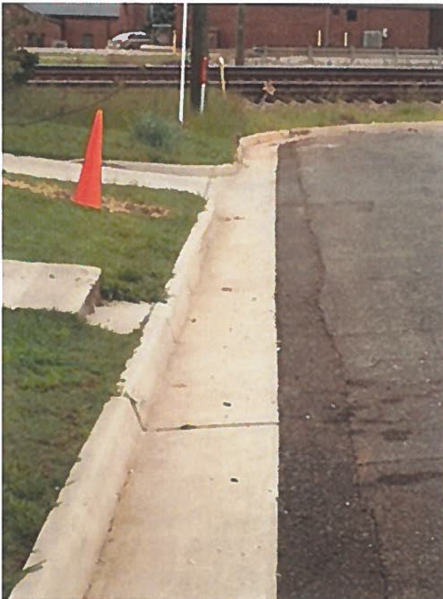
Existing curb and gutter along Broad Street (flow goes toward railroad tracks)
