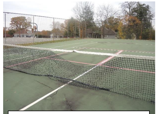
Broken Nets and cracked court surface
