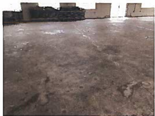
Floor: Aging condition of existing concrete slab
