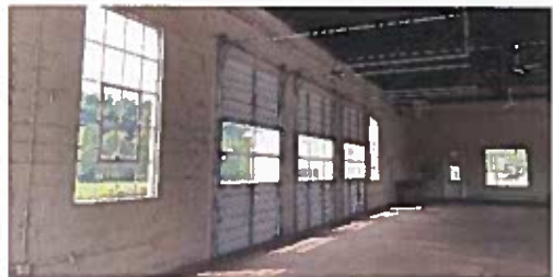
Cooling: Ceiling fans and rolling doors are used for summer cooling
