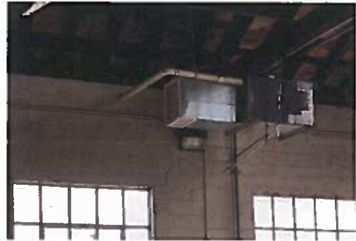
Heating: Corner mounted heating unit
