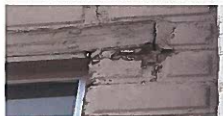
Walls: Painted concrete block walls need repairs and painting in some locations.
