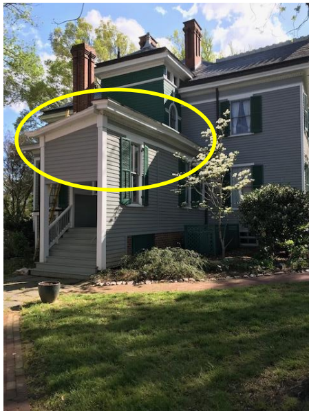
FIGURE 1 – The two-level roofs above the mansion's porch and kitchen is highlighted. They are metal roofs whose rusted-out portions and poorly-applied membrane are allowing water inside the structure and that water is leaking through underneath to the porch. Without intervention, the interior of the house will show that leak, as well.
