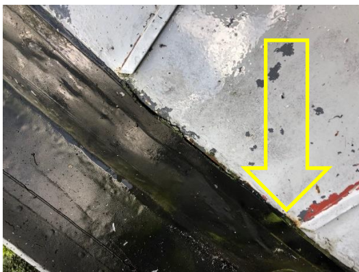
FIGURE 5 – The rubber membrane is separating from the metal roof and this will lead to more problems in the absence of roof and membrane replacement.
