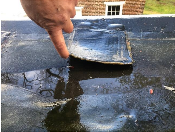
FIGURE 3 – Patches on the rubber membranes are failing and allowing water in. Also, the membranes themselves are coming detached from the roof and allowing a great deal of water in addition to the water that the rusted-out portion of the roof is allowing.
