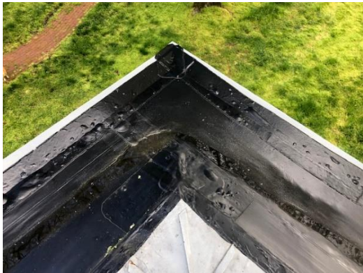
FIGURE 4 – The rubber membrane is above, not below the metal roof. According to several roofing professionals, this is a result of improper application many years ago and will surely lead to roof leaks. The professionals say that the membrane needs to be laid underneath the metal portion of the roof.
