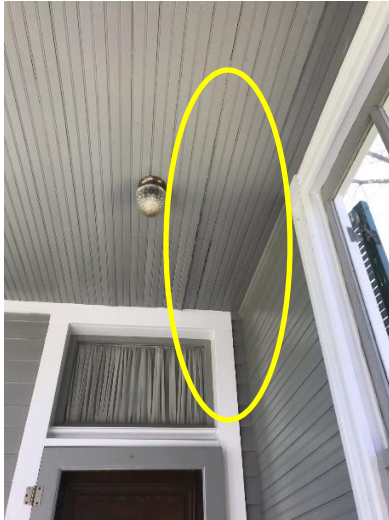
FIGURE 2 – Roof leaks are causing water to run through the ceilings above the mansion’s side porch and interior kitchen. The water is dripping through and causing damage to the porch ceiling. Thankfully, however, the water is not yet dripping through into the house over the kitchen.
