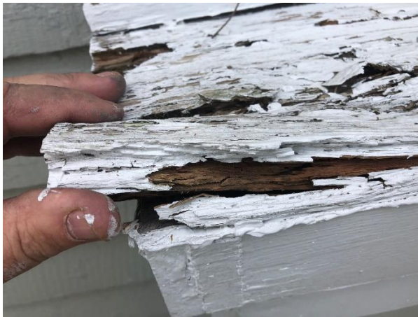
FIGURE 7 – Pigeon's perch damage
