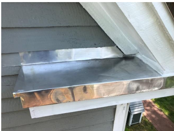
FIGURE 8 – Restored pigeon's perch with metal flashing to prevent a recurrence of the problem
