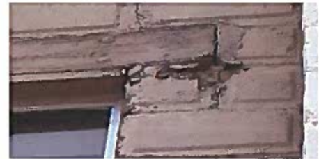
Walls: Painted concrete block walls need repairs and painting in some locations.
