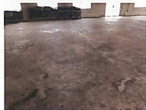
Floor: Aging condition of existing concrete slab
