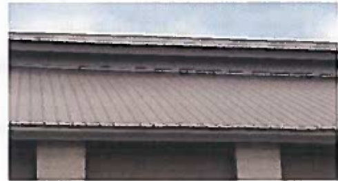
Roof: Metal roof needs some repairs and additional flashing
