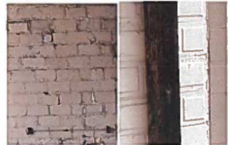
Walls: Concrete block walls are uninsulated and paint is beginning to age and crack. Decorative block wall is an interesting existing design feature.
