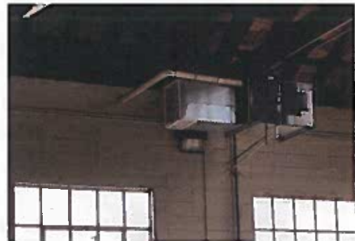
Heating: Corner mounted heating unit
