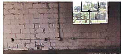
Electric: Existing outlets, conduits and breaker boxes
