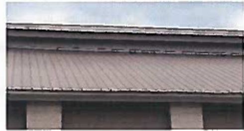
Roof: Metal roof needs some repairs and additional flashing
