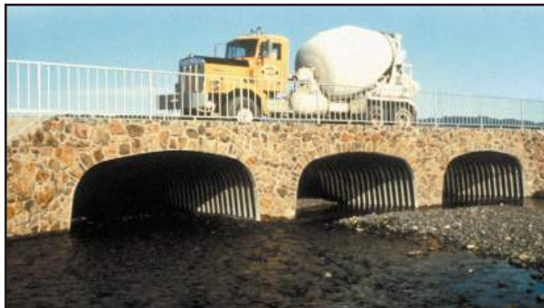
Aluminum Box Culvert - county road bridge
