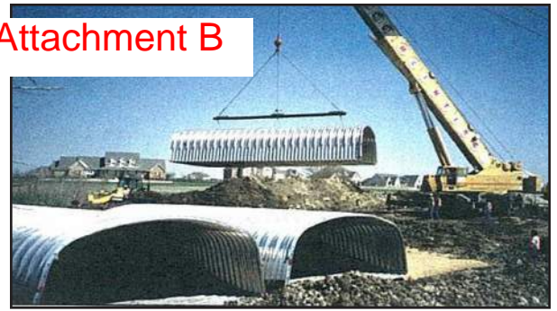
Aluminum Box Culvert - multi-cell installation
