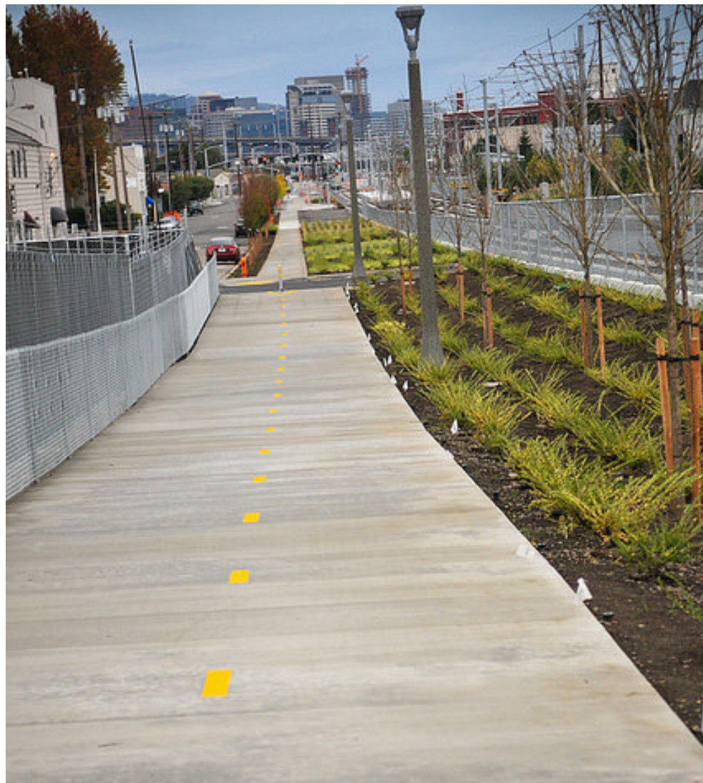
Left: This is an example of a raised multi-use path that features a vegetation buffer. This accommodates both cyclists and pedestrians as there is just this two-way facility.
