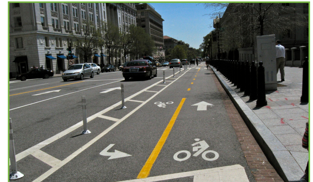
Right: Urban cycle track with larger buffer between bicyclists and vehicular traffic
