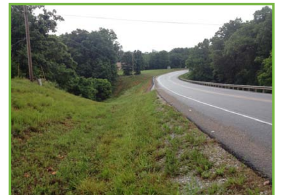
Looking east at Lancashire Rd. land bridge where steep cross slopes will be challenging for trail development.
