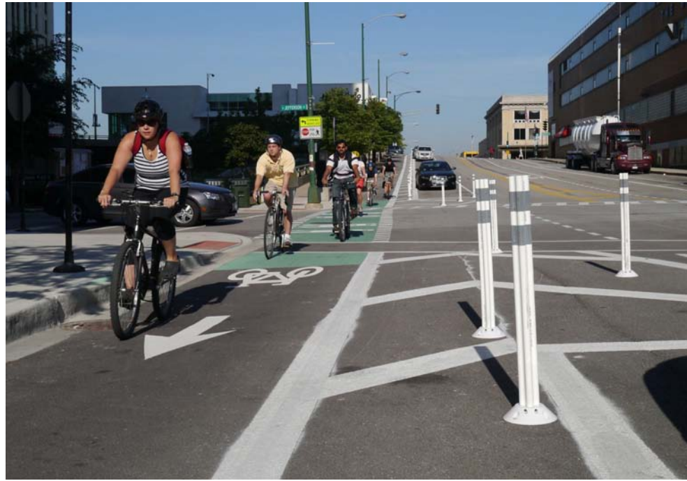
Left: An example of a one-way cycle track is shown. The proposed Towncenter Promenade could feature a striped buffer and bollards as one alternative.
