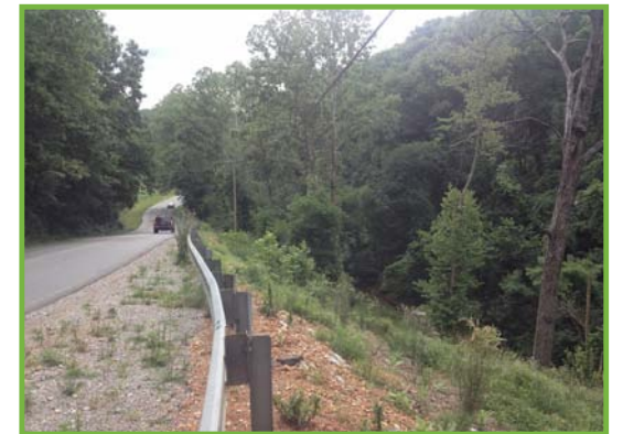
In some areas, trails are not feasible, such as this steep ravine off Riordan Rd. near Kenton Ln.
