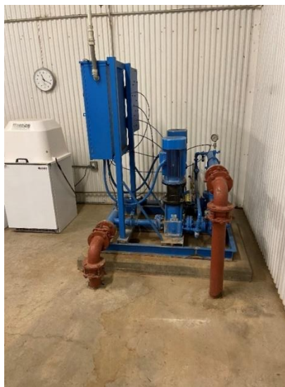
WASHWATER BOOSTER PUMP SKID WITHOUT BLADDER TANK
