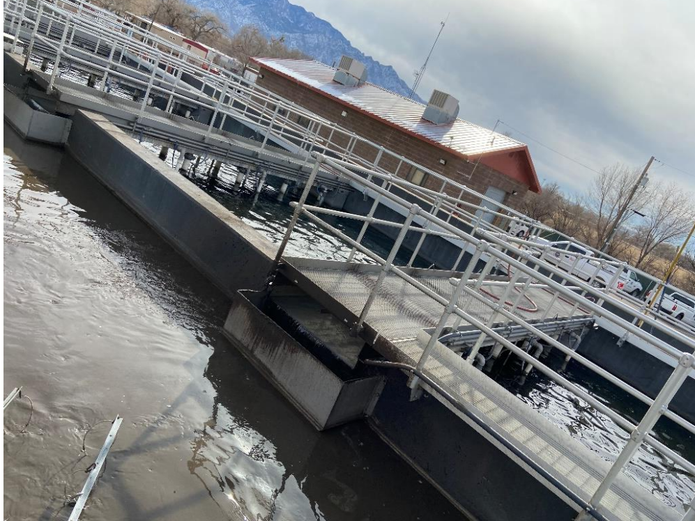
VIEW OF SOUTH AERATION BASIN
