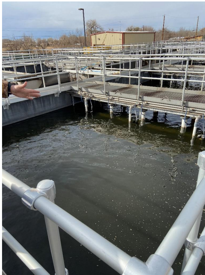
VIEW OF CLARIFIER AND WALKWAY BRIDGE
