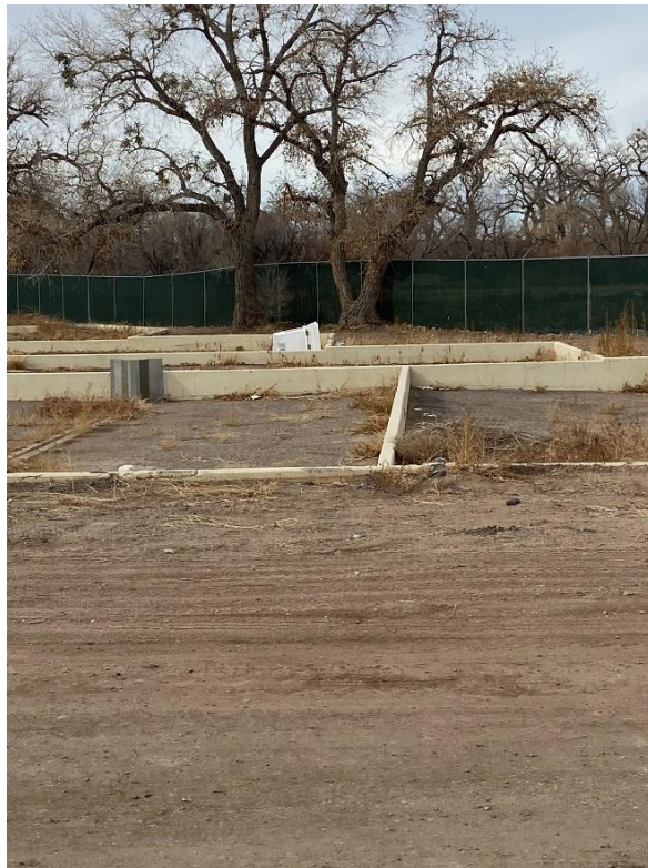
SLUDGE DRYING BEDS – EAST SECTION
