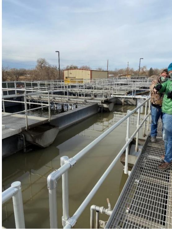
VIEWS OF FERMENTER BASIN AND RAS INLETS FROM AERATION BASINS. ANAEROBIC BASIN IS ON WEST SIDE OF FERMENTER BASIN.
