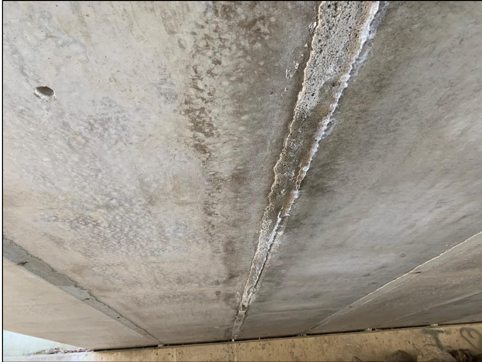
Photo 5: Efflorescence and minor beam cracking 2 nd joint from upstream fascia beam, below the sidewalk.
