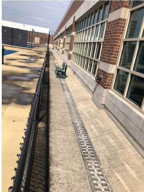
Photograph No. 3: Drain Tile Along East Side of Courts
