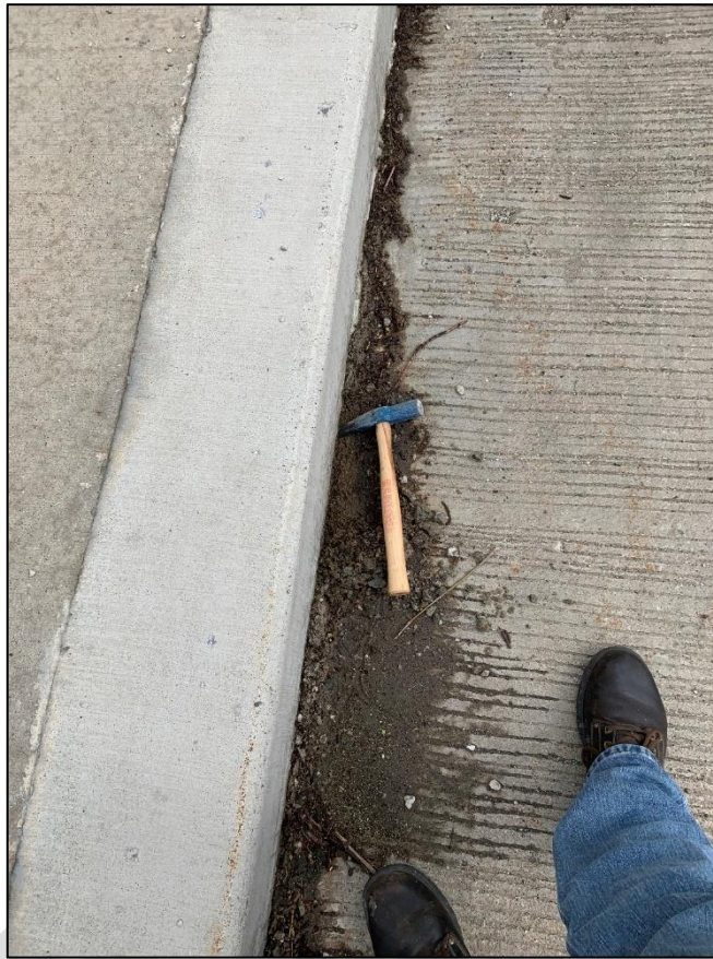
Photo 3: Sidewalk deterioration along deck joint.
