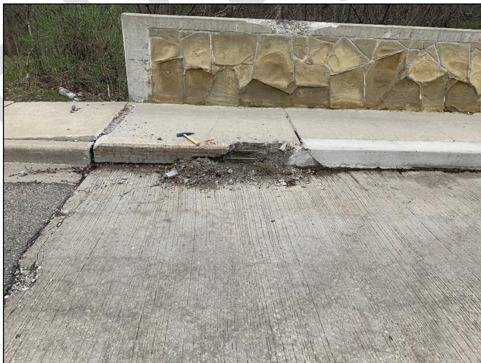
Photo 4: Exposed reinforcement in sidewalk
