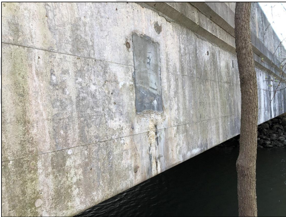
Photo 6: Efflorescence and cracking in post-tensioned grout pocket.
