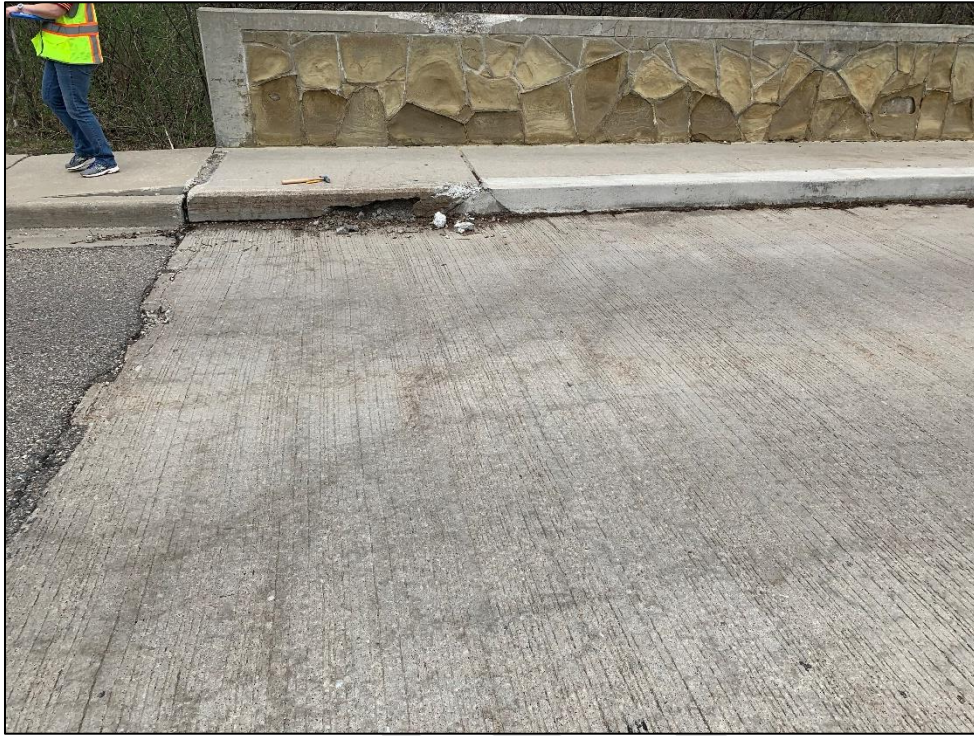
Photo 1: Deck cracking, sidewalk deterioration, and railing spalls in Northwest quad.
