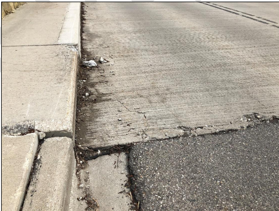
Photo 2: Deck cracking and sidewalk deterioration in Northwest quad.
