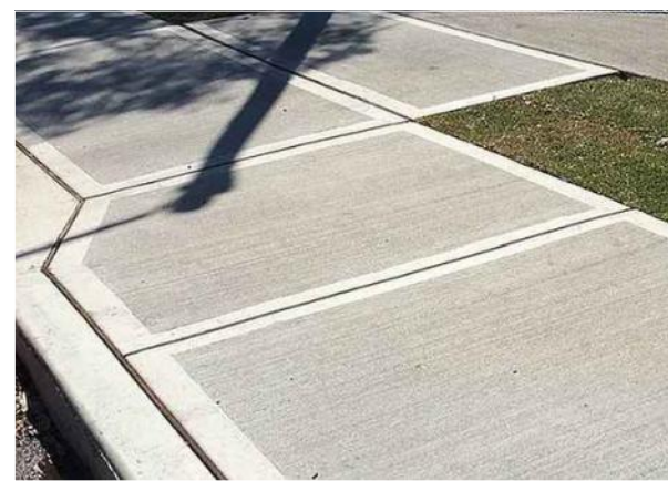
A decorative pedestrian concrete walk BROOM FINISH WITH 3" SMOOTH TROUPEL FINISH BETWEEN SCORING
