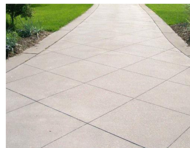
I specialty pavement concrete saw scored 45 degrees
