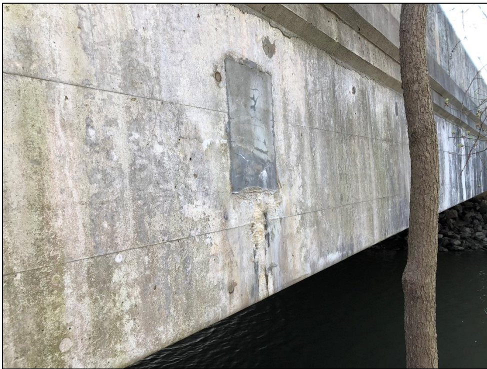
Photo 6: Efflorescence and cracking in post-tensioned grout pocket.
