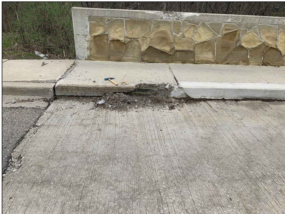
Photo 4: Exposed reinforcement in sidewalk
