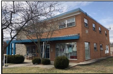
Above – The cantilevered metal awning of the Hennessey Building at 240 Main St. is appropriate for a 1960 commercial building.
