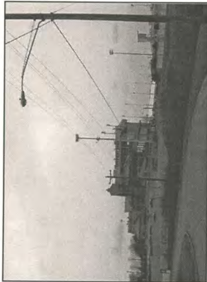
FIGURE 4 Cell Tower Attached to Light Pole
