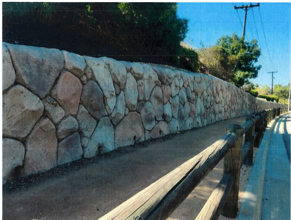
Figure 2. Boulder Face Soil Nail Wall
