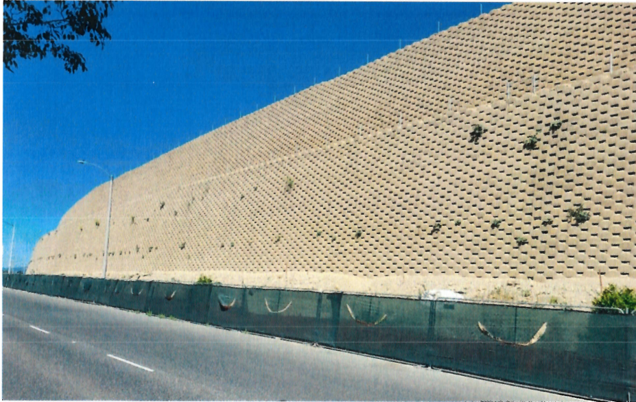
Figure 5. MSE (Gravity) Retaining Wall
