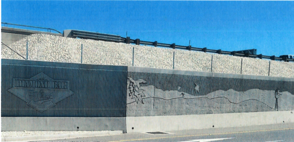
Figure 3. Form Pour Concrete Soil Nail Wall
