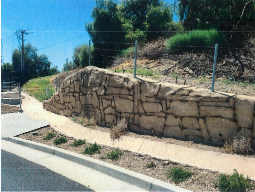
Figure 1. Rock Face Soil Nail Wall
