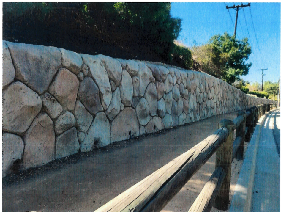
Figure 2. Boulder Face Soil Nail Wall
