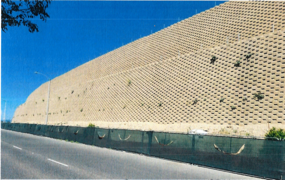
Figure 5. MSE (Gravity) Retaining Wall
