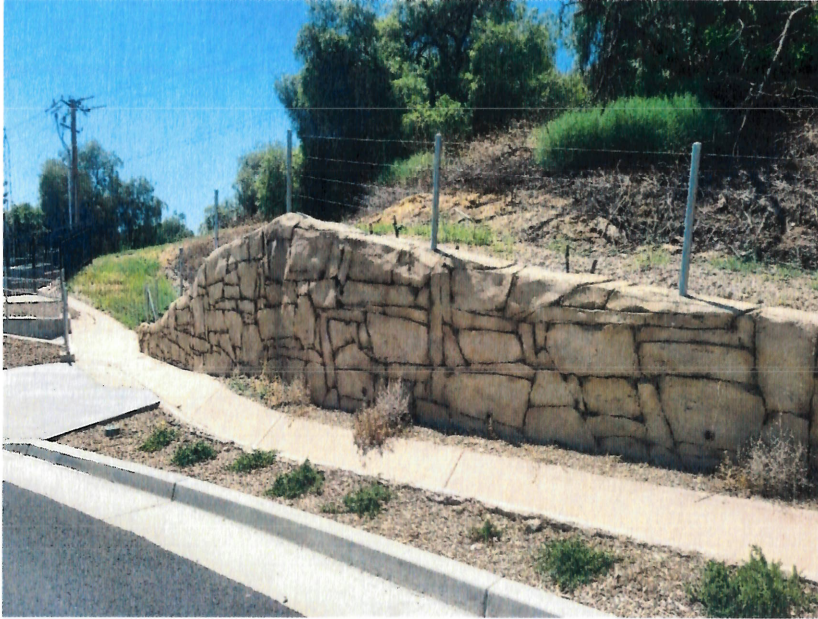
Figure 1. Rock Face Soil Nail Wall
