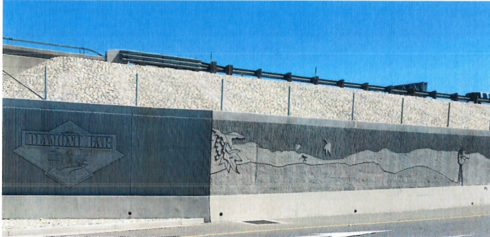
Figure 3. Form Pour Concrete Soil Nail Wall
