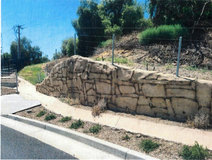
**Figure 2. Boulder Face Soil Nail Wall**
