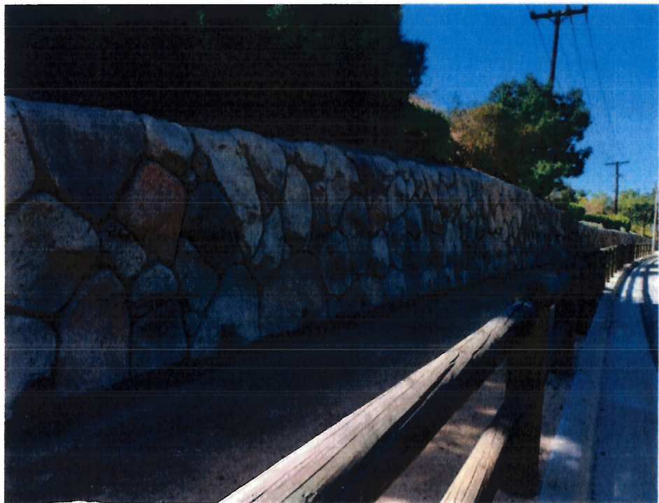
Figure 2. Boulder Face Soil Nail Wall
