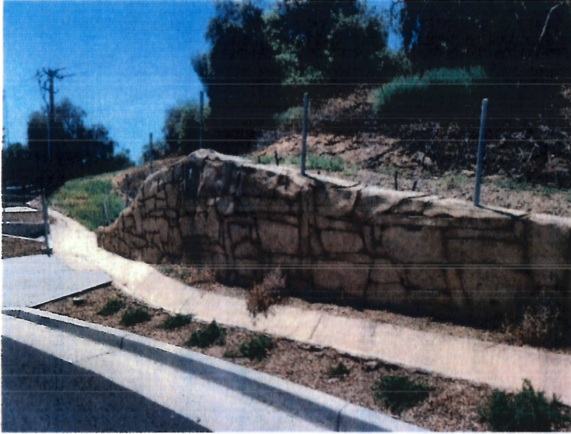
Figure 1. Rock Face Soil Nail Wall
