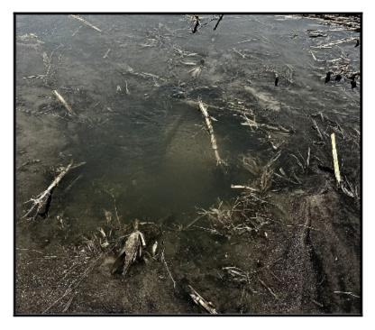
On the March 13th site visit the field was no longer flooded, and we were able to identify several additional blowouts/suck holes in the Main Tile. We note that the tile has less than 1 foot of cover (depth of soil over the top of the pipe). The distance between the lowermost and uppermost tile blowouts observed is approximately 900 feet.
