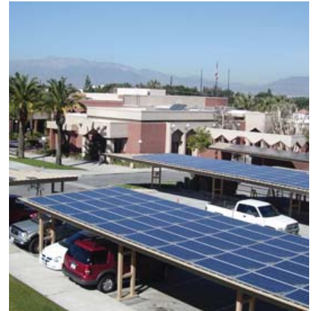
Solar shade structure
