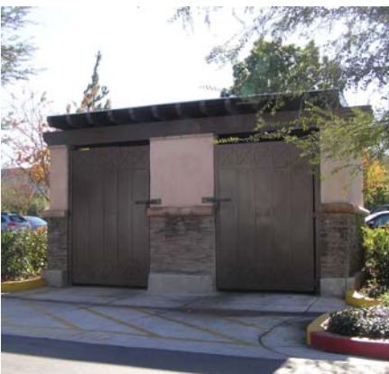
Trash enclosures must be covered and should compliment the design of the adjacent architecture
