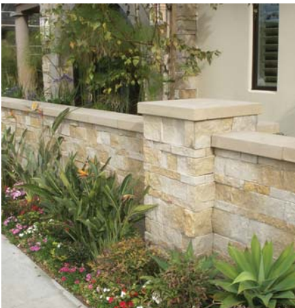
Fences and walls less than three feet are appropriate in front yards
