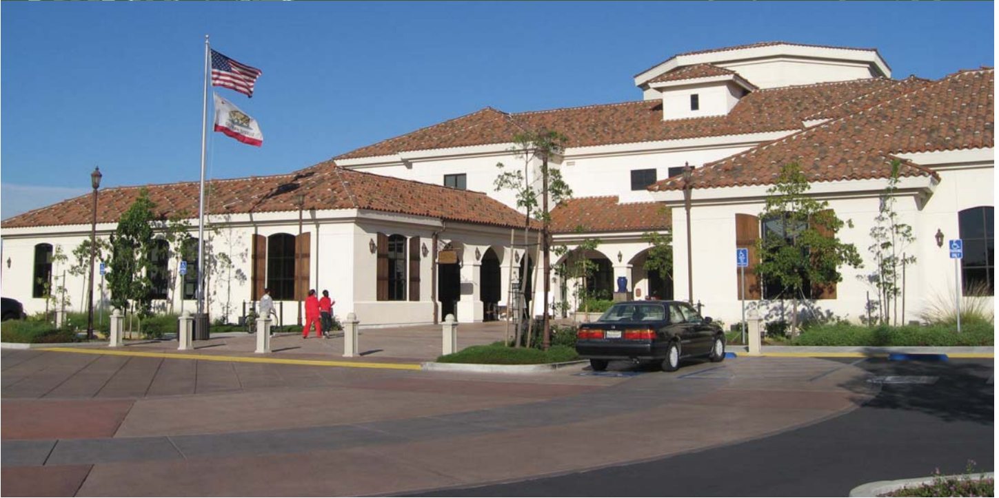
The library has a desirable architectural character
