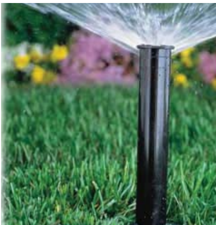
Irrigation systems should have efficient flow and coverage
