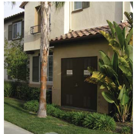
Utility areas should be integrated into building design
