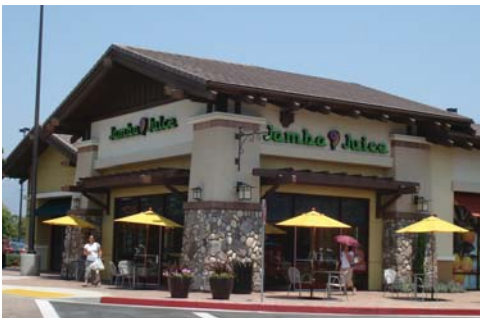
Overhangs and eaves accentuate entrance
