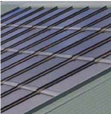
Solar panels transfer sunlight into energy
