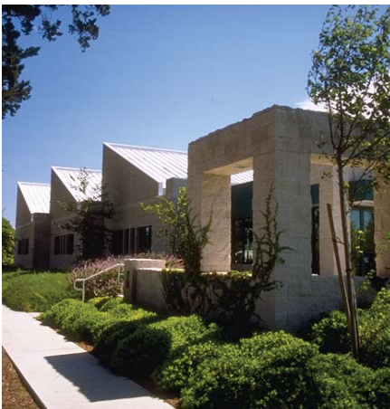
Pedestrian walkway identifies building entrance
