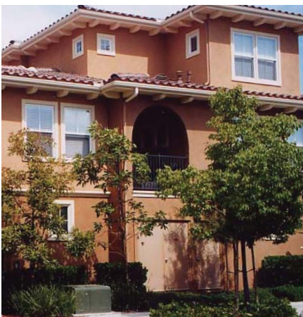
A mechanical room has been incorporated into the overall building design
