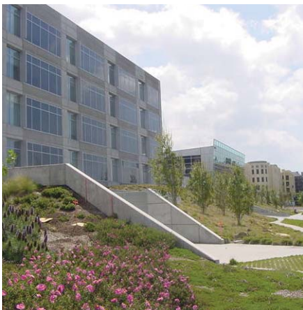
Landscape berms decrease impact of loading areas and mechanical equipment
