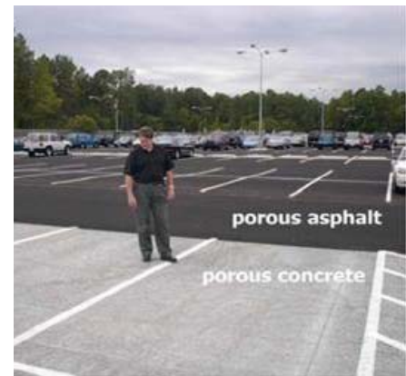
Porous concrete has a higher reflectance than porous asphalt
