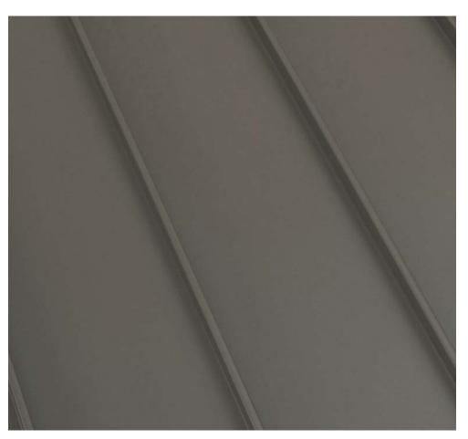
METAL ROOFING -STANDING SEAM TYPE MR-1
