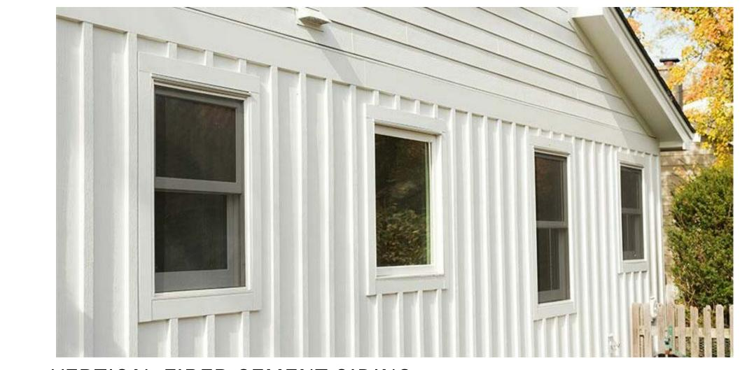
VERTICAL FIBER CEMENT SIDING -BOARD AND BATTEN SIDING TYPE VC-1
